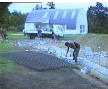
Re-laying the foundation blocks After the first were kicked over
