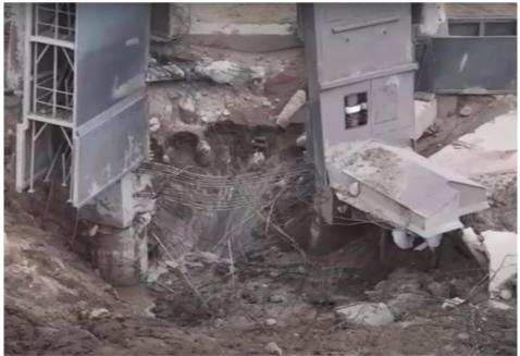
The damage to the base of the structure shows the sheer power of the 36 engines. The rocket literally dug a pit beneath the pad before it managed to overcome gravity and rise into the sky.
