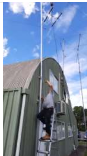
Ian pulling up the multiband antenna.
