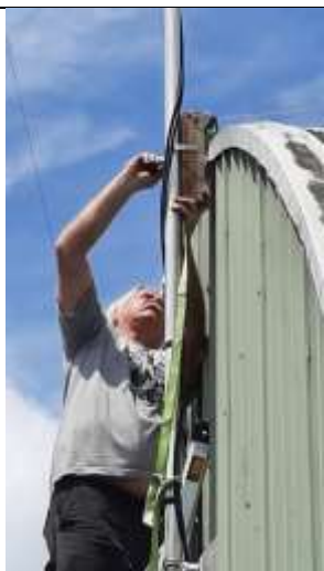
Cable support in position, Ian tightens the stainless-steel clamp
