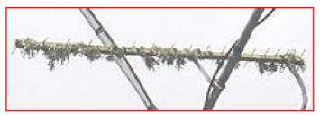
Problem What is the best way to remove moss from an antenna with a wooden boom? Unfortunately this one is too high to reach. We have thought of transmitting high power but this may result in self-destruction of the above item. Application of RF to antennas in moderate amounts hinders moss growth... Answers to the editor (Note:-this is not my antenna!!)
