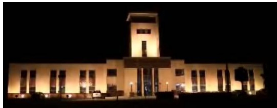
The VOA transmitter building.
