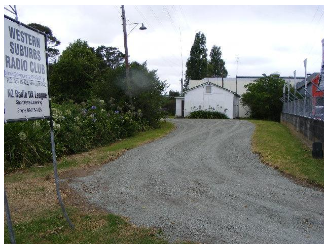
The new metal drive.
