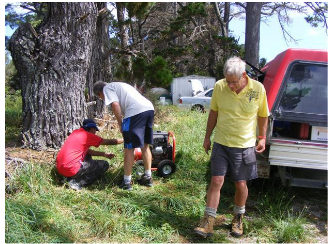
Work on the Generator.
