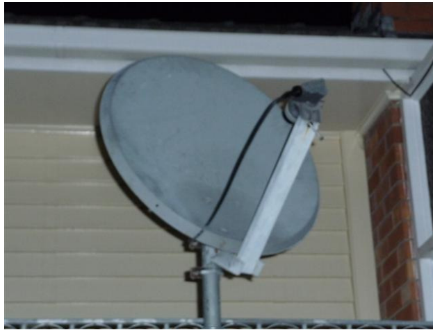
Typical Satellite Dish Capable of receiving Free to Air Channels Aligned to the Optus D1 Satellite
