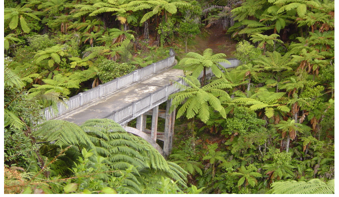
Bridge to Nowhere amongst the ferns
