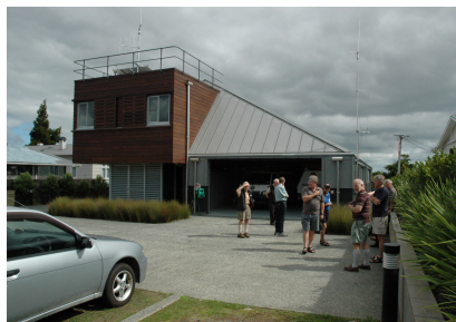
Rear View of the CD Headquarters
