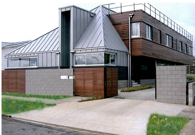
Waitakere Civil Defence Headquarters
