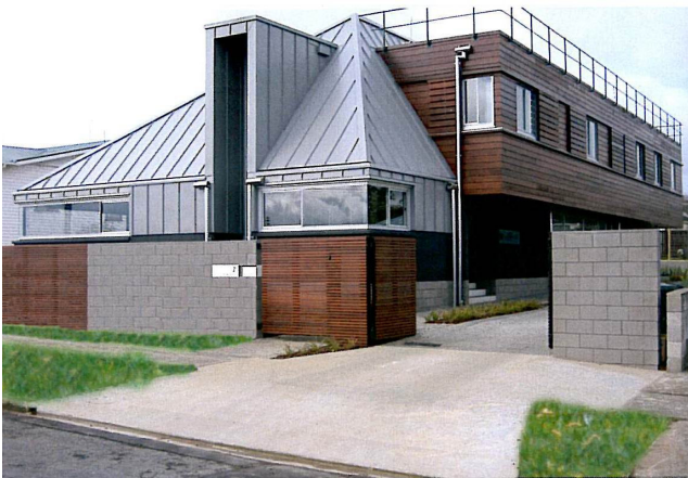
Waitakere Civil Defence Headquarters
