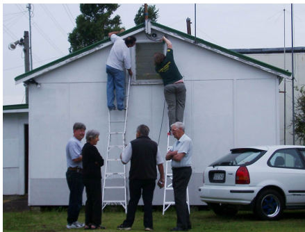
Installing the Antenna Pole and cable
