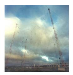
HR 2/4/0.5 is a five band curtain antenna with a frequency range of 9.5 to 17.9MHz.
