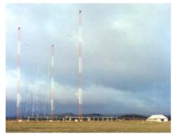
HR 2/2/1 is a four band dipole curtain antenna with a frequency range of 5.95 to 12.05 MHz.
