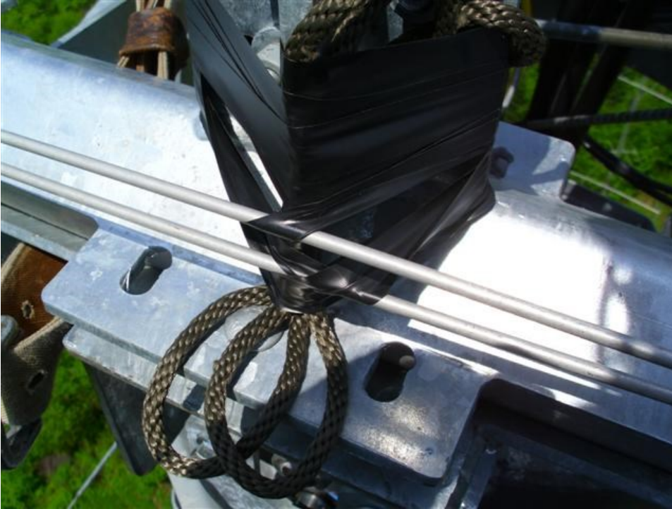
Figure 588 Stretching phasing line around boom truss
