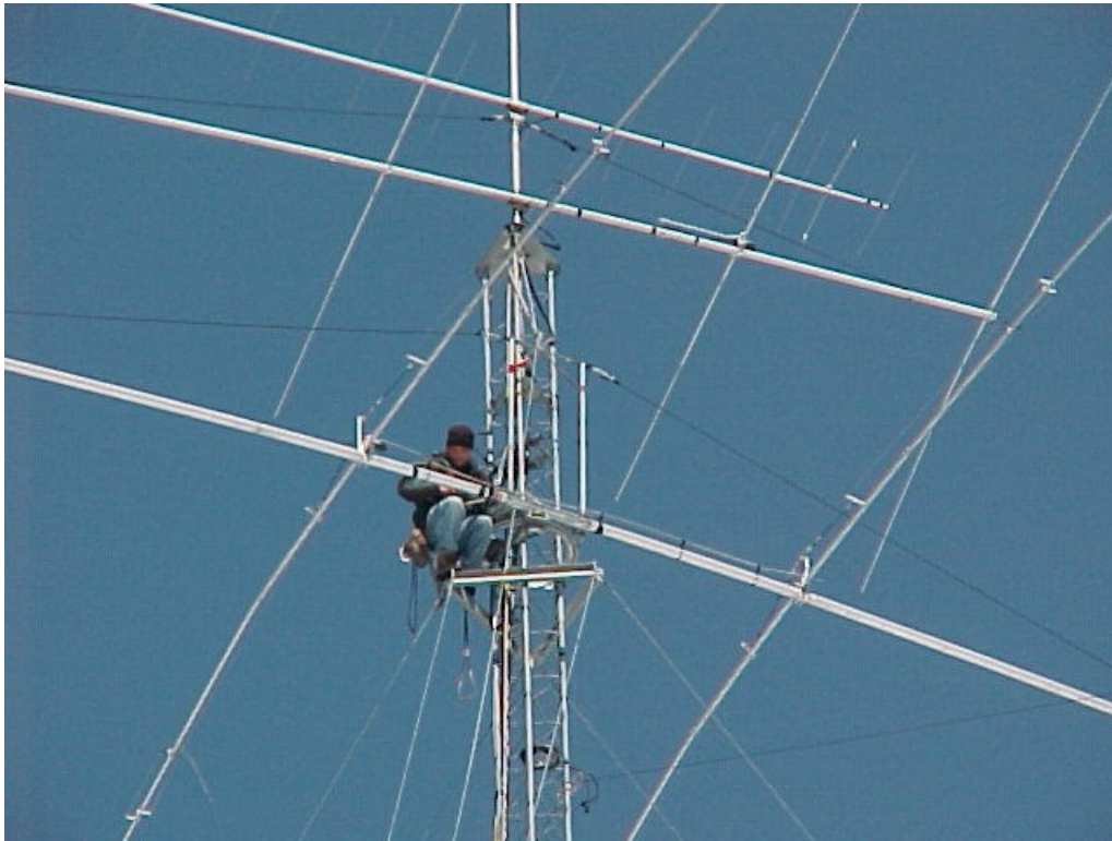
Figure 322 Rigging the top 40m.
