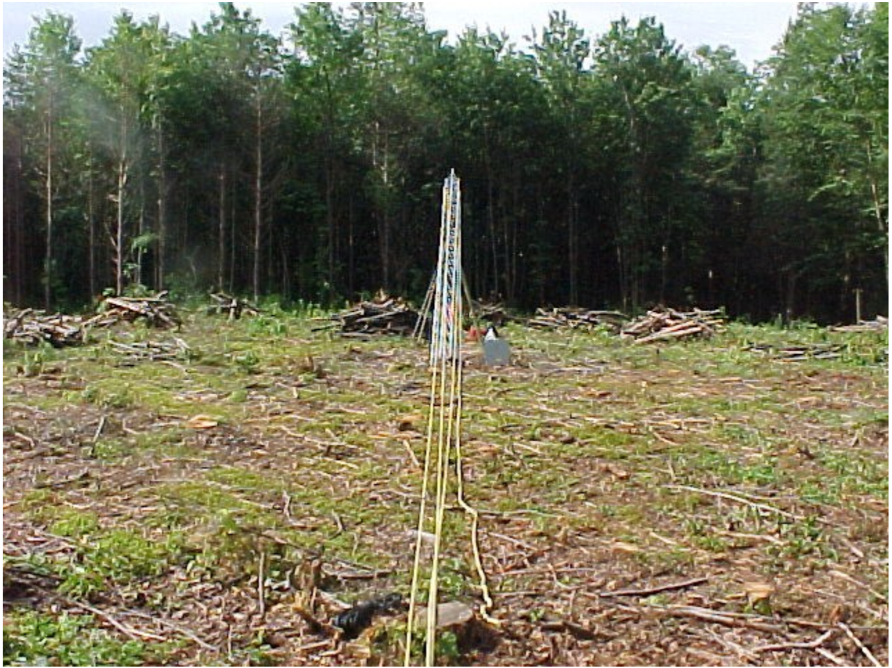
Figure 276 Putting up Gin Pole tower going up.
