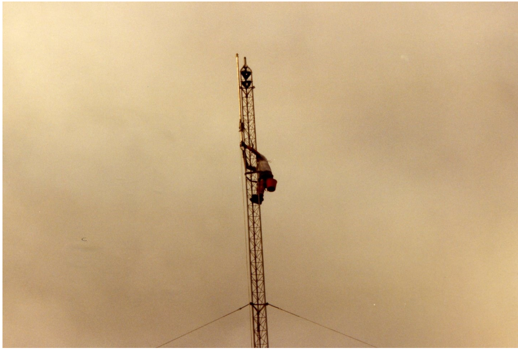
Figure 107 last section in place, now for last guys.
