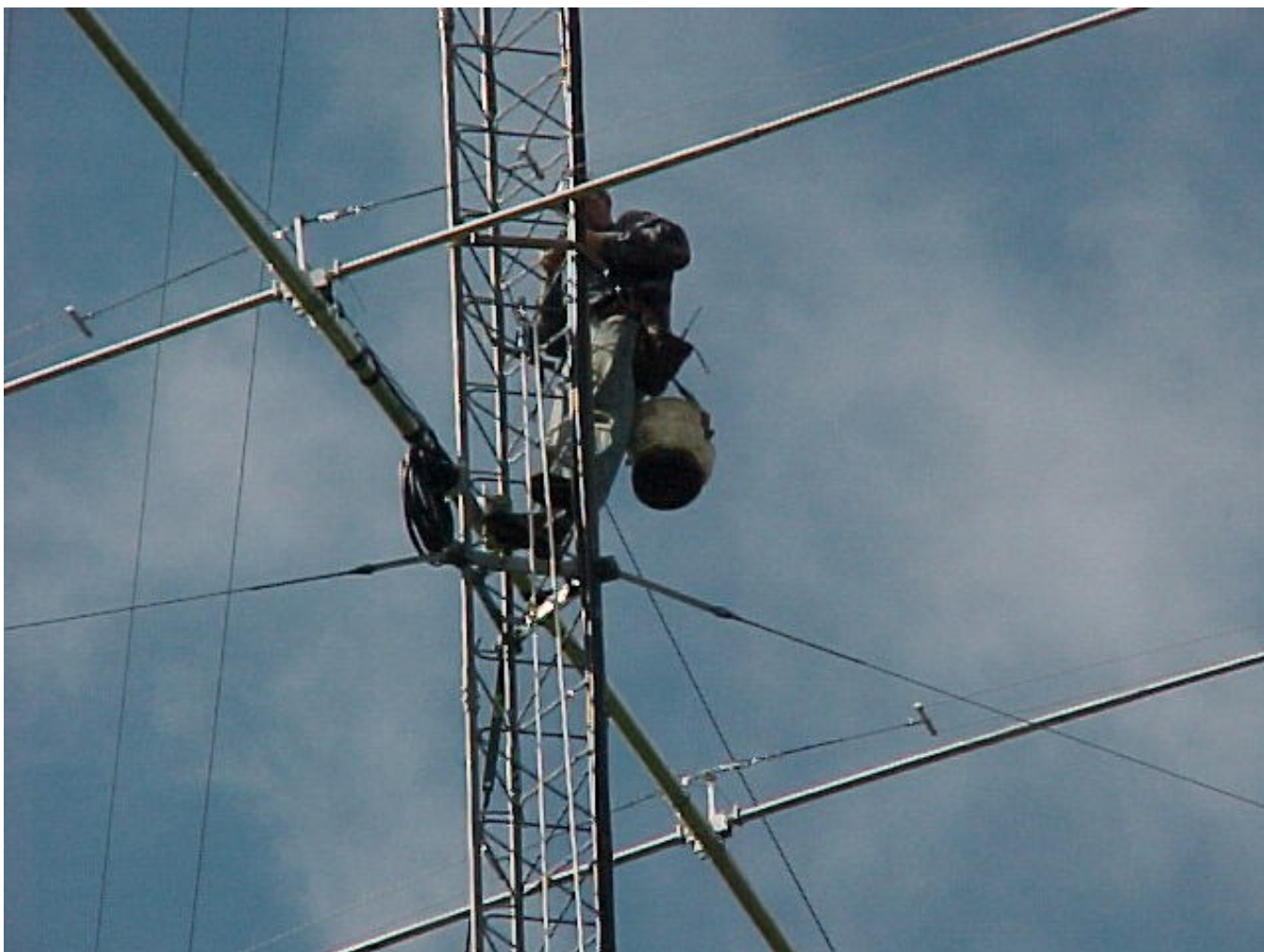
Figure 177 Finishing up boom braces.
