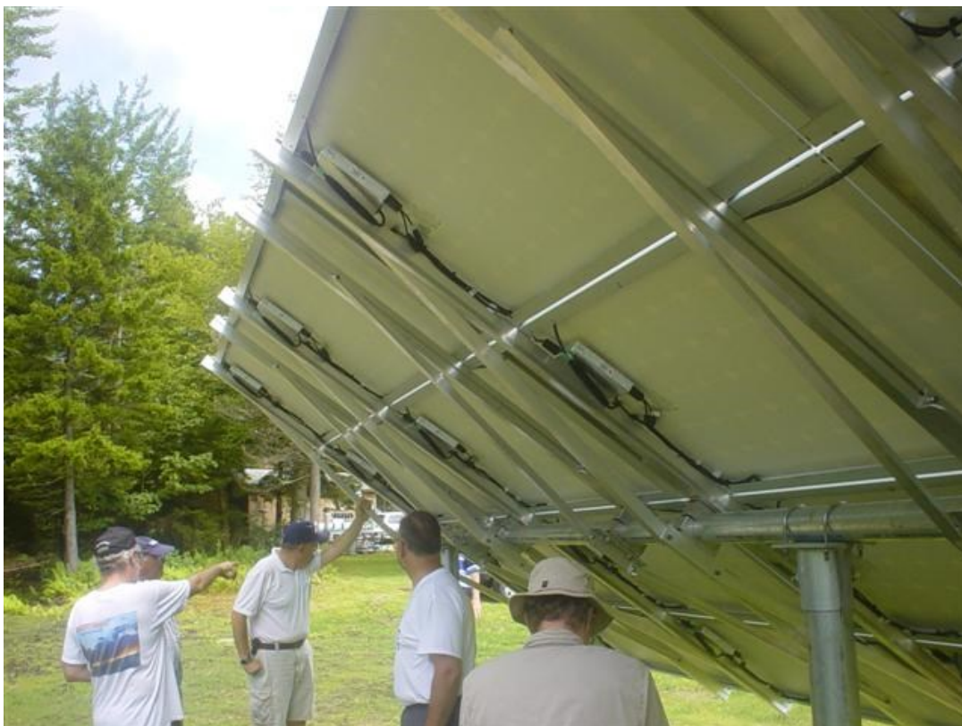
Figure 526 A look behind the solar array showing the micro inverters.
