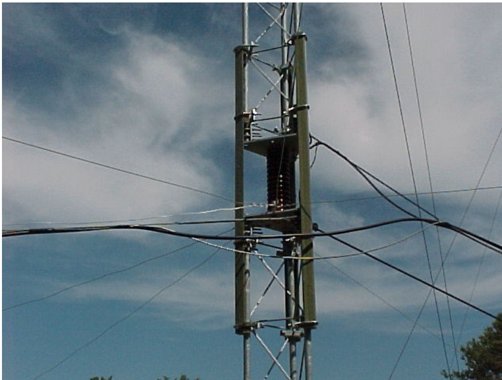
Figure 331 The new strongbacks in place.
