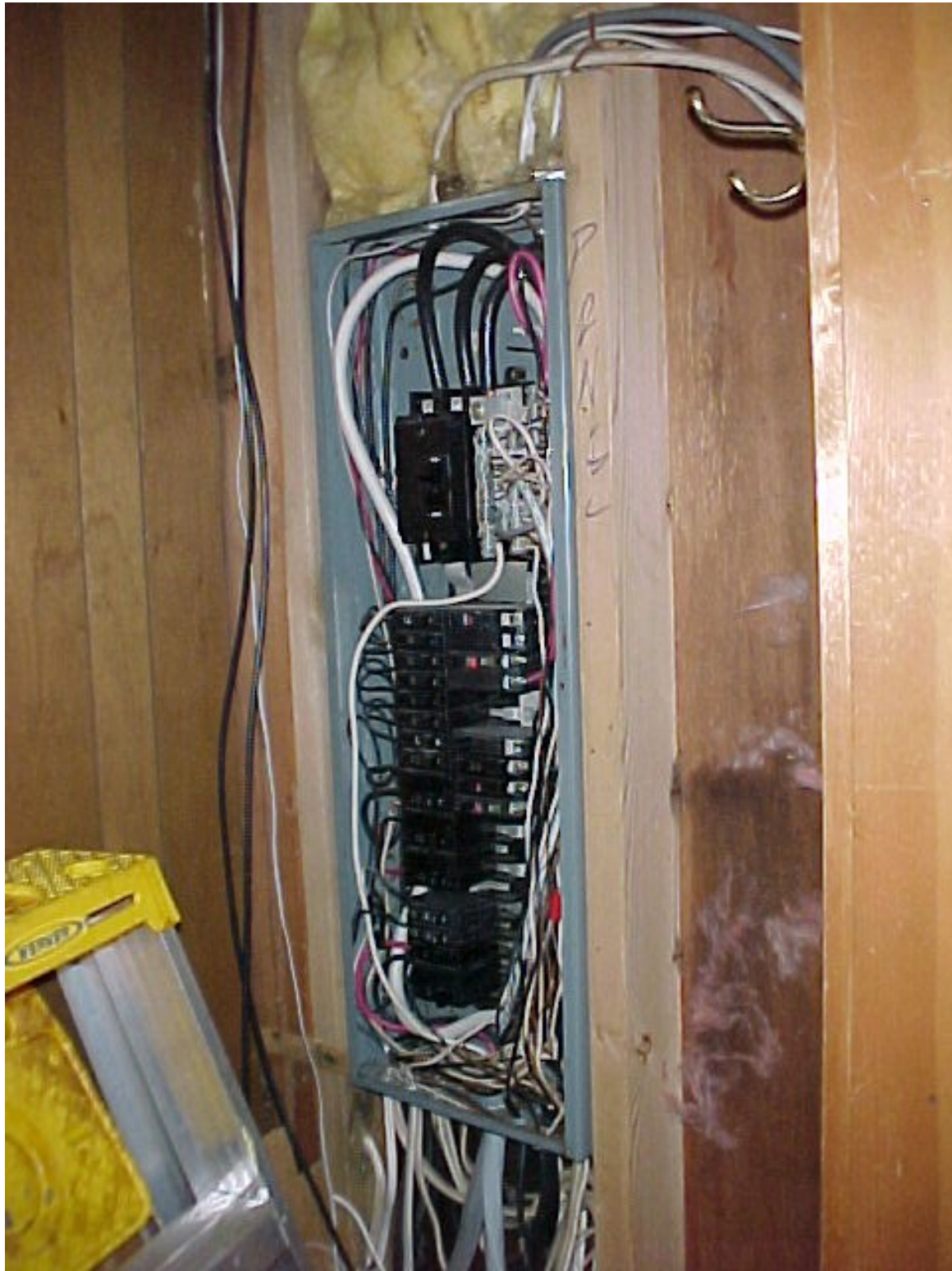
Figure 482 The main panel before wiring in the generator.
