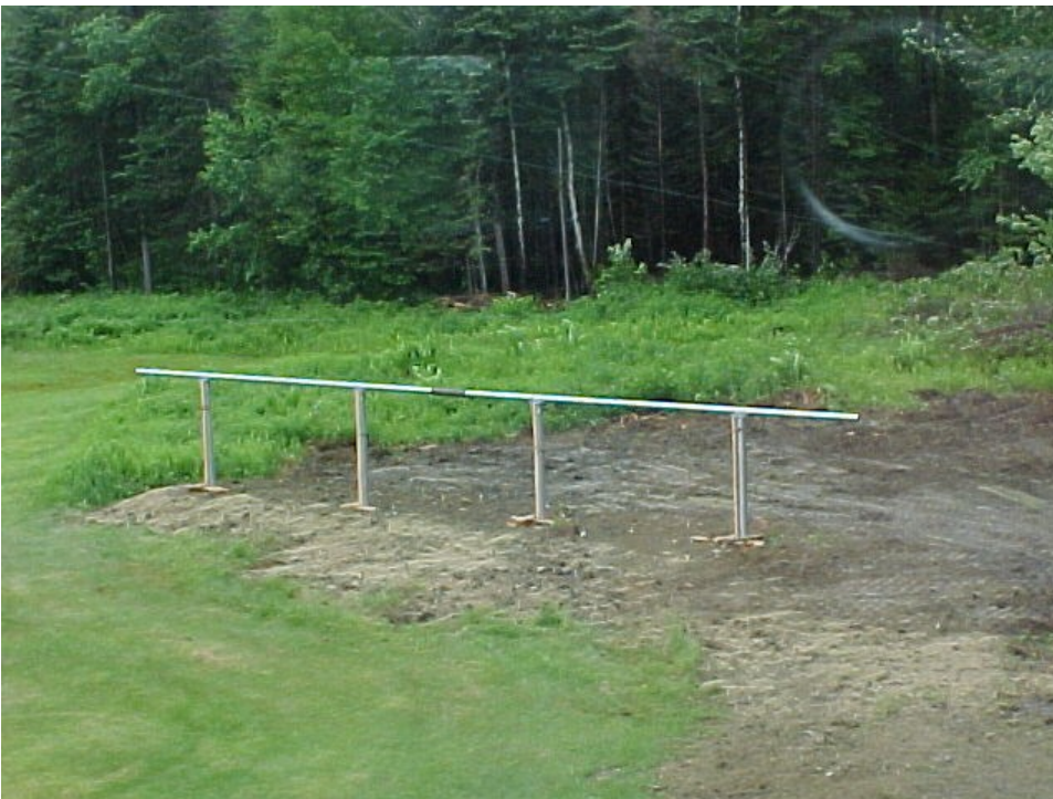
Figure 512 This the the completed mounting frame for the solar system
