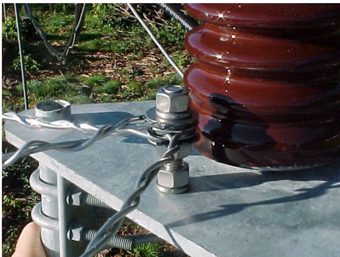
Figure 295 Radial connection points.
