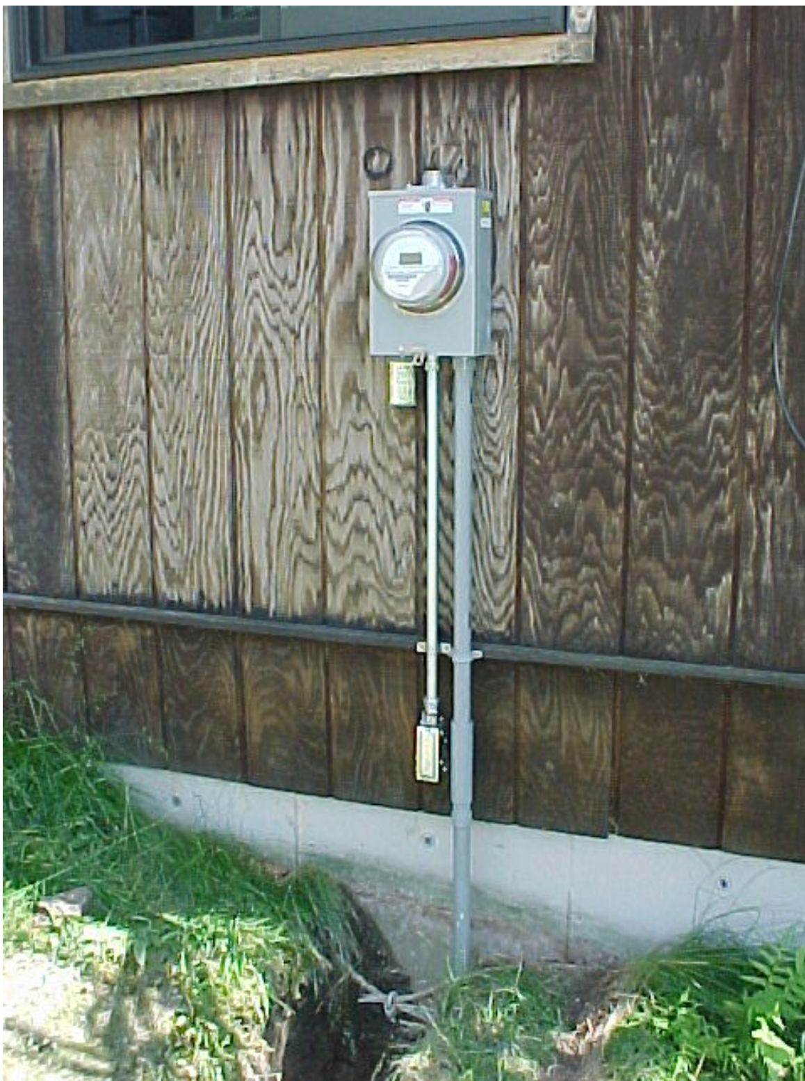
Figure 508 Another meter just for the solar system on the other end of the house
