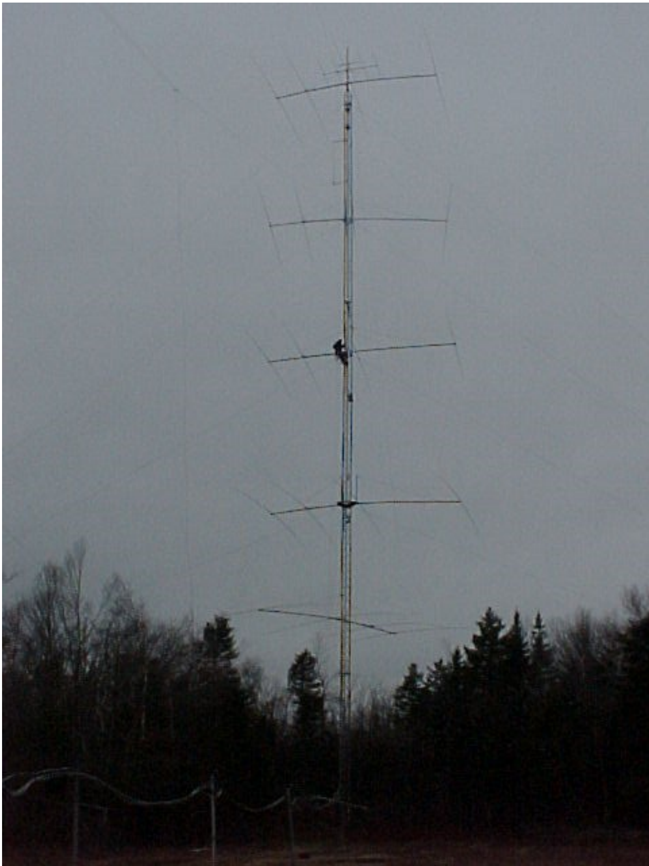
Figure 412 Finishing up the 90' 20m4dx. The 120' one just above it is the one that was put up last Friday.
