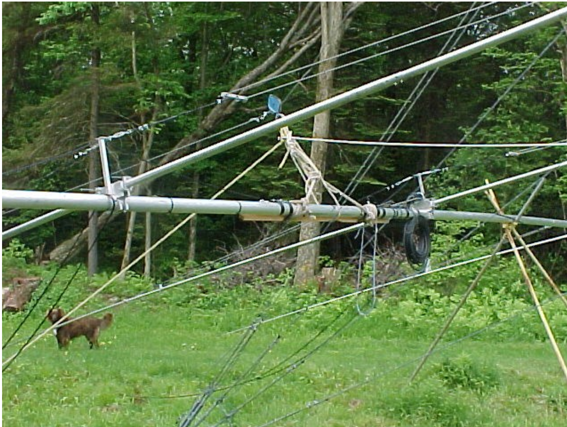
Figure 193 Rigging the 40M4LLDD to tram.
