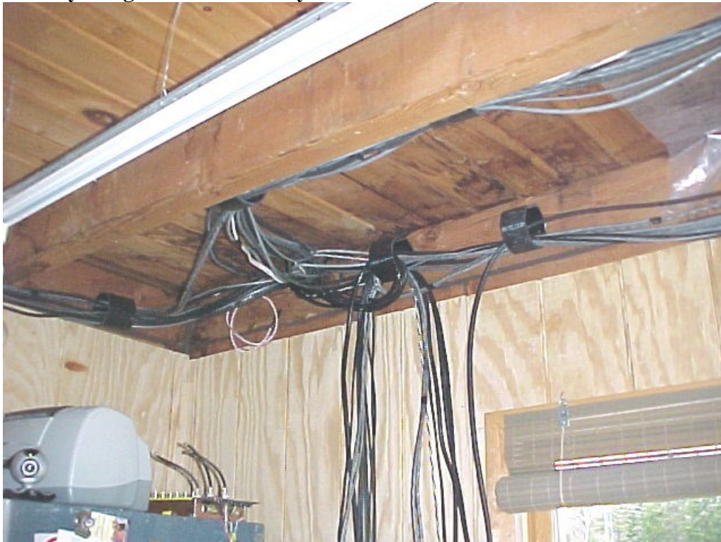
Figure 251 Cleaned up wire entrance.
