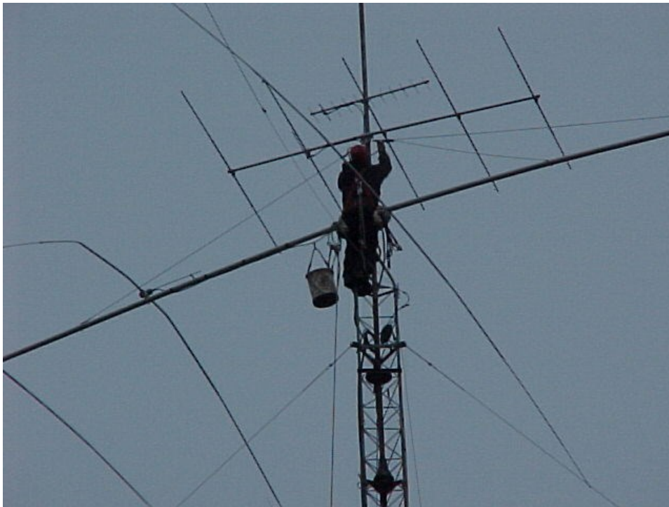
Figure 410 Andrew getting started at 150'. Note the extra boom truss rope on the right side, that is to stop the boom from fluttering in light winds.
