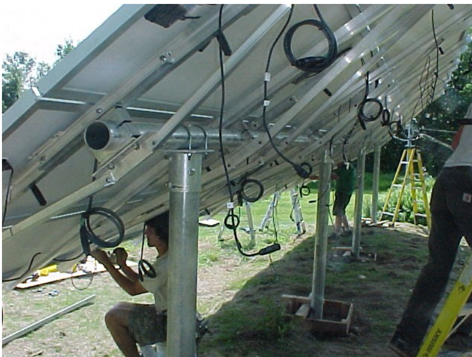
Figure 515 Wiring solar array
