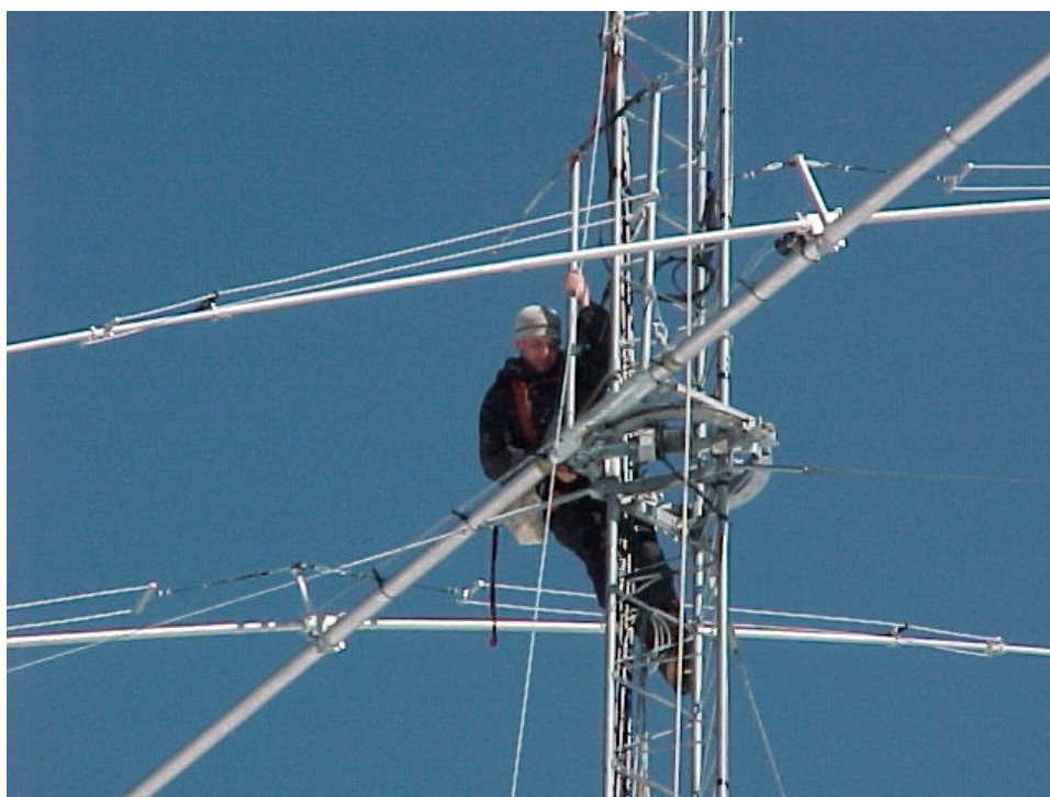
Figure 390 Level it out and bolt it down.
