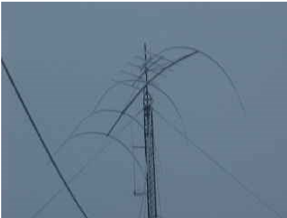
Figure 353 Top 20m before wind came up and broke the elements.
