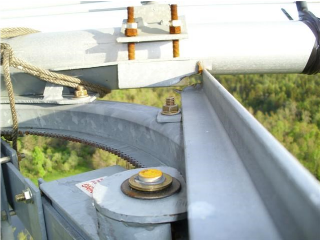
Figure 585 Broken top TIC ring
