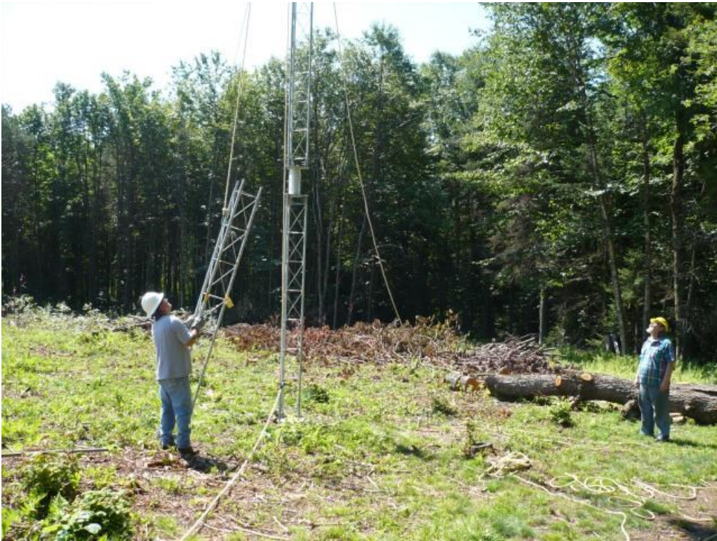
Figure 289 Section heading up.
