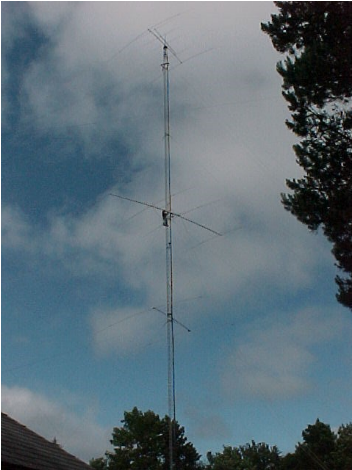
Figure 175 Antenna off tram wire, swinging around tower.
