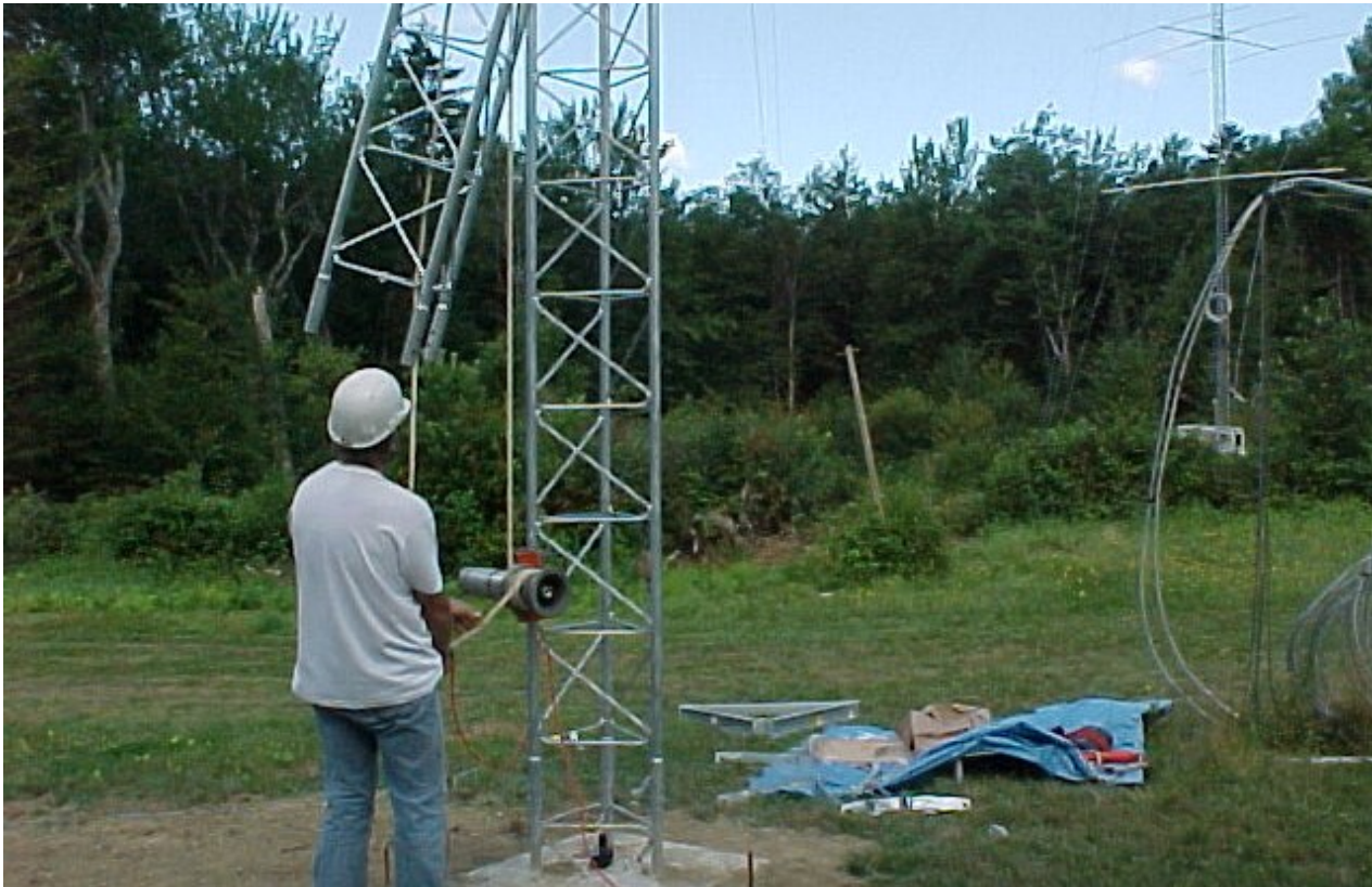
Figure 123 KC1XX raising Rohn 55 section
