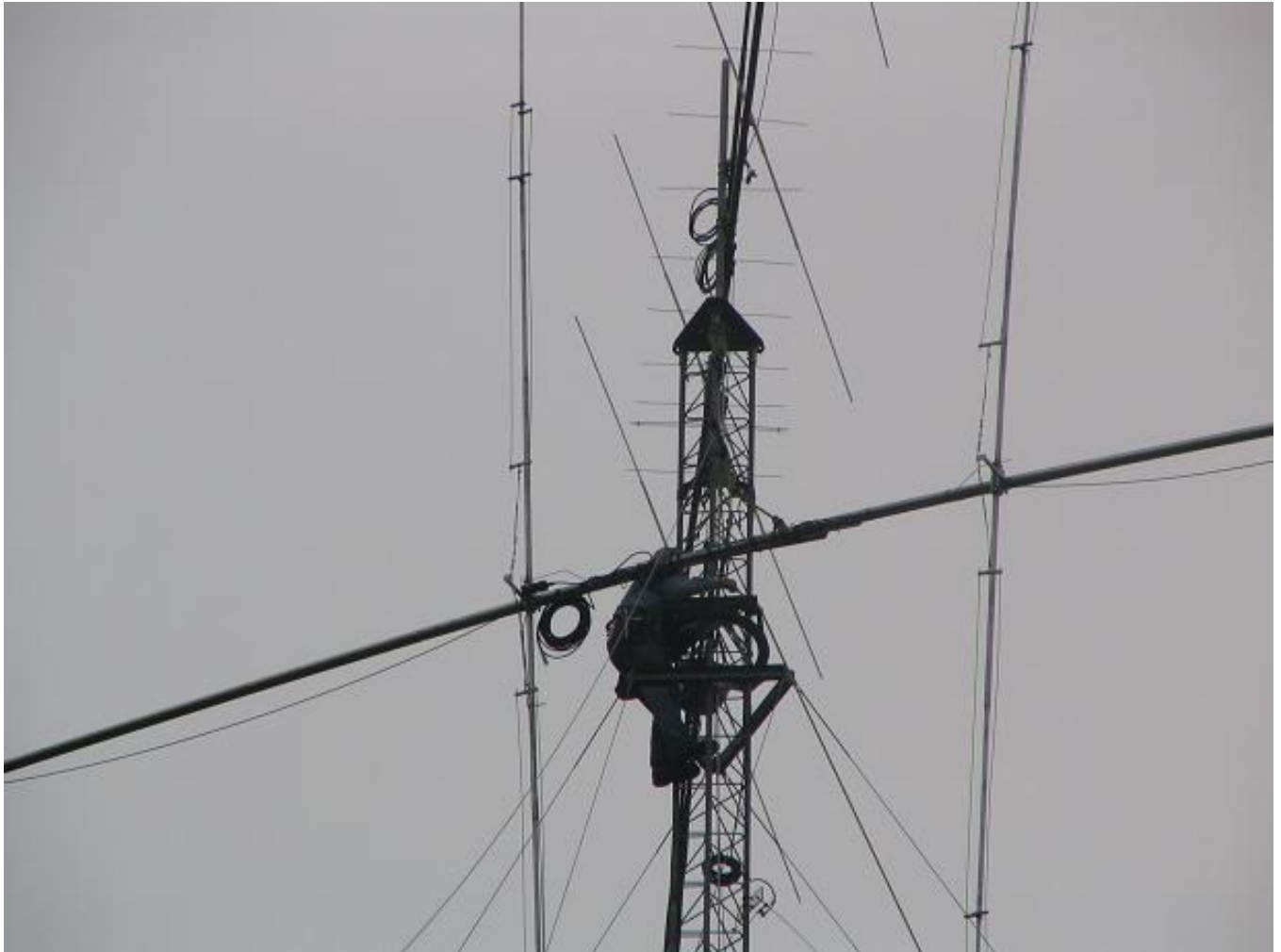
Figure 203 Flipping the 10m beam on its side made room to level it off.
