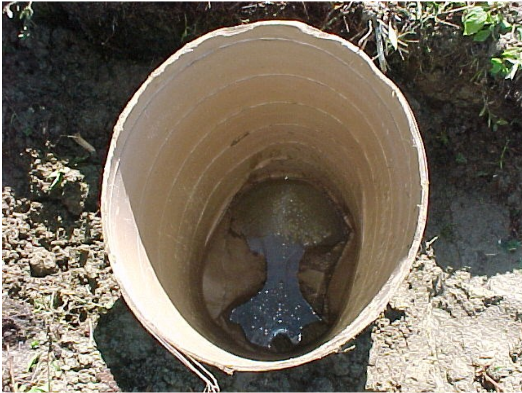
Figure 506 Wet Sonotubes don't work very well
