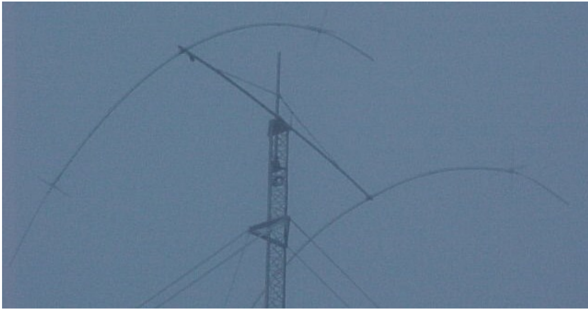
Figure 131 Ice builds up even faster at 180'.
