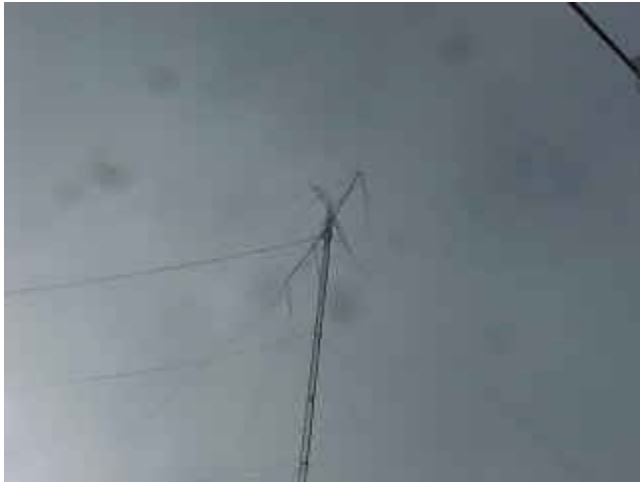
Figure 362 The top of the 180' tower after the wind, 10m and 2m are both broke.
