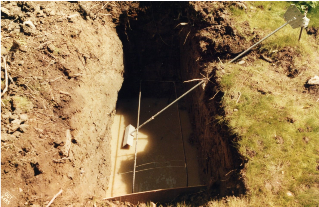
Figure 12 Anchor hole
