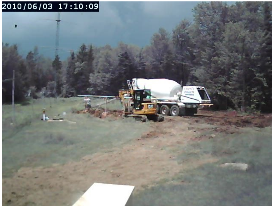
Figure 510 pouring foundations
