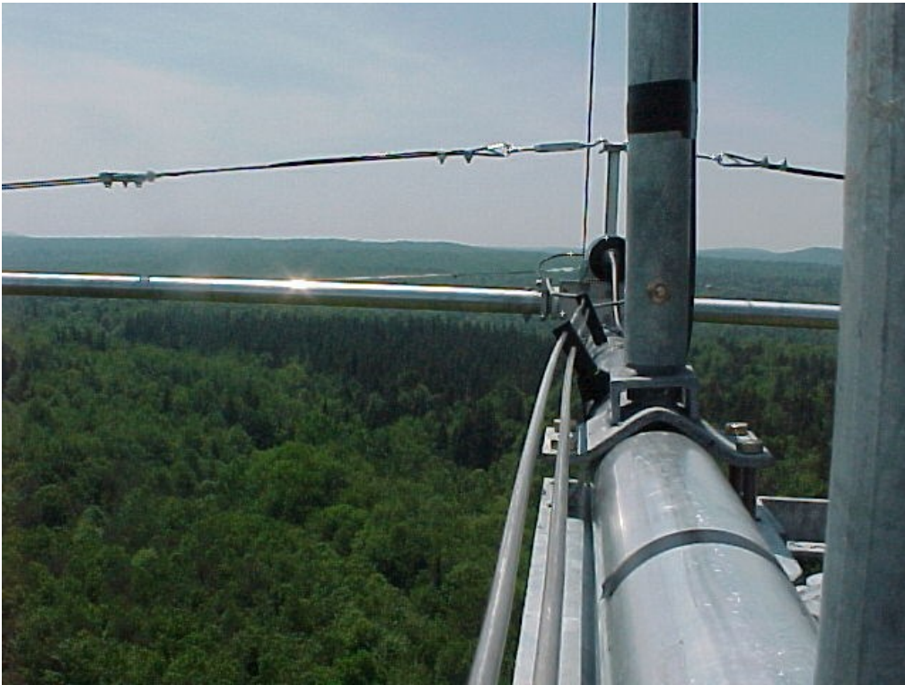
Figure 211 phasing line and boom struts final.
