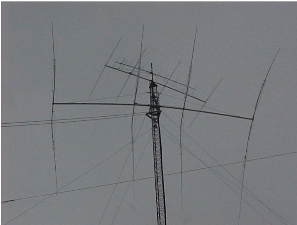
Figure 316 Top 40m with ice and wind, slightly crooked elements.
