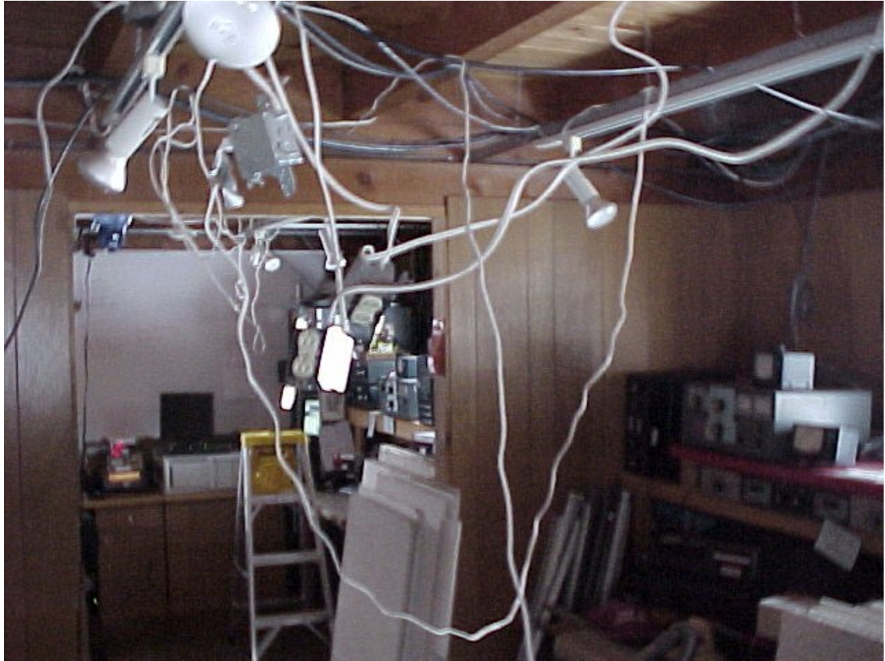
Figure 237 Old wiring.
