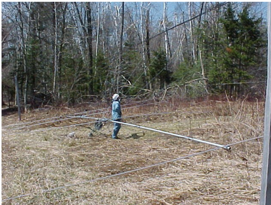
Figure 407 The 20m4dx ready to go up using the top guy wire as a tram.
