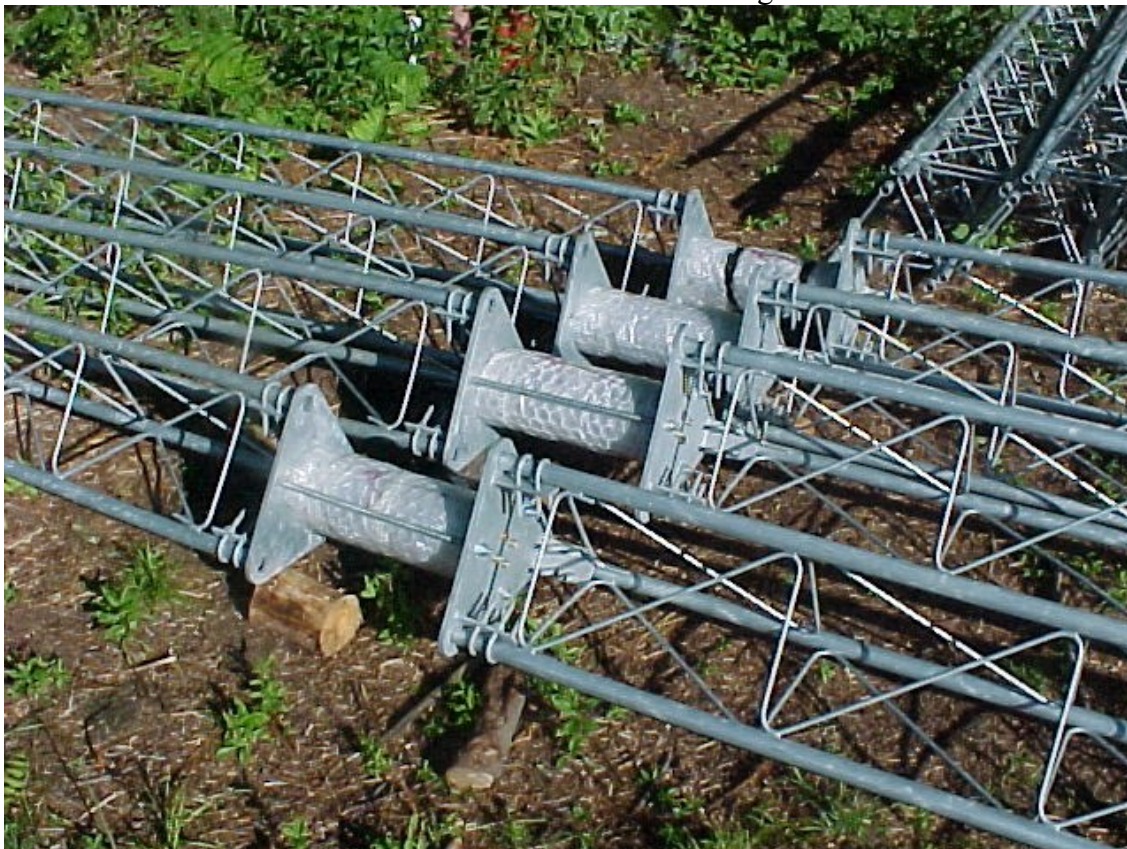
Figure 274 Insulators all in place with rods.
