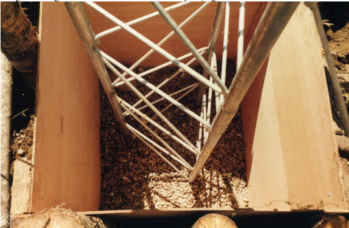
Figure 13 Base hole with gravel and short base section
