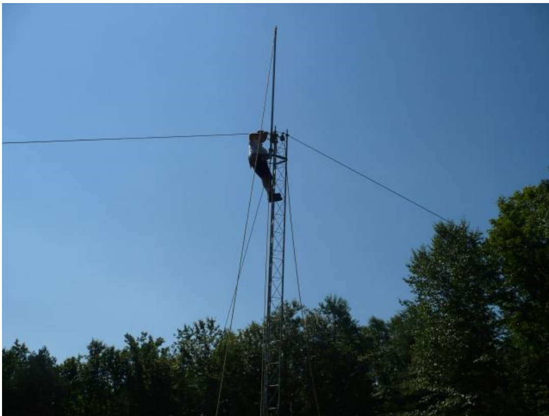
Figure 288 Installing Gin Pole.
