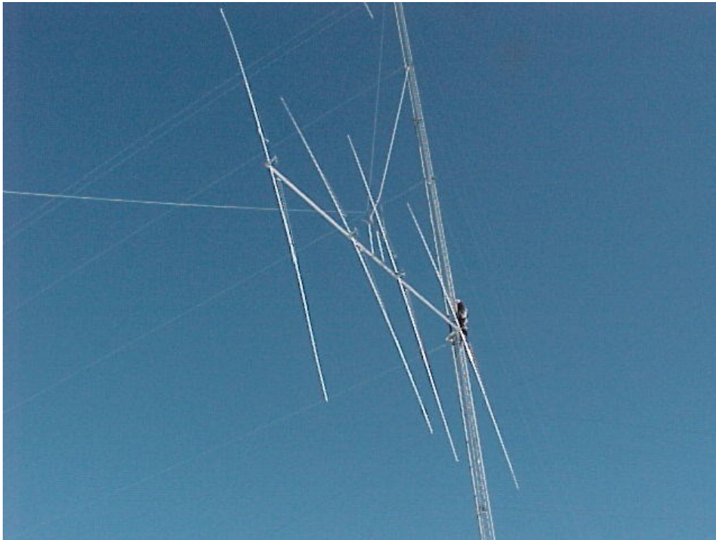
Figure 385 The sling was too tight and tipped the antenna all the way up sideways, I'm not the only one that can do that I guess.
