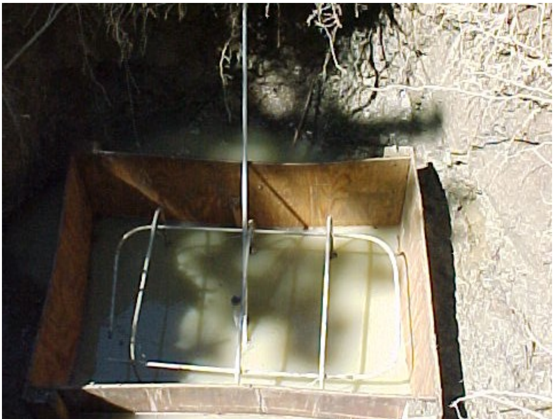
Figure 122 Anchor form and rebar
