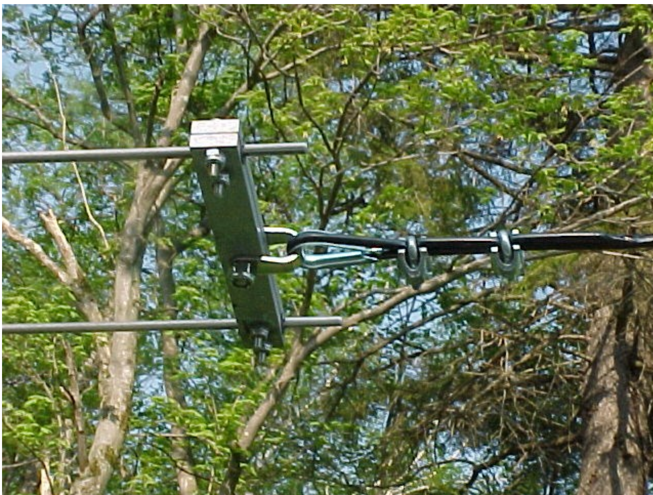
Figure 265 Modified shorting bar and attachment.
