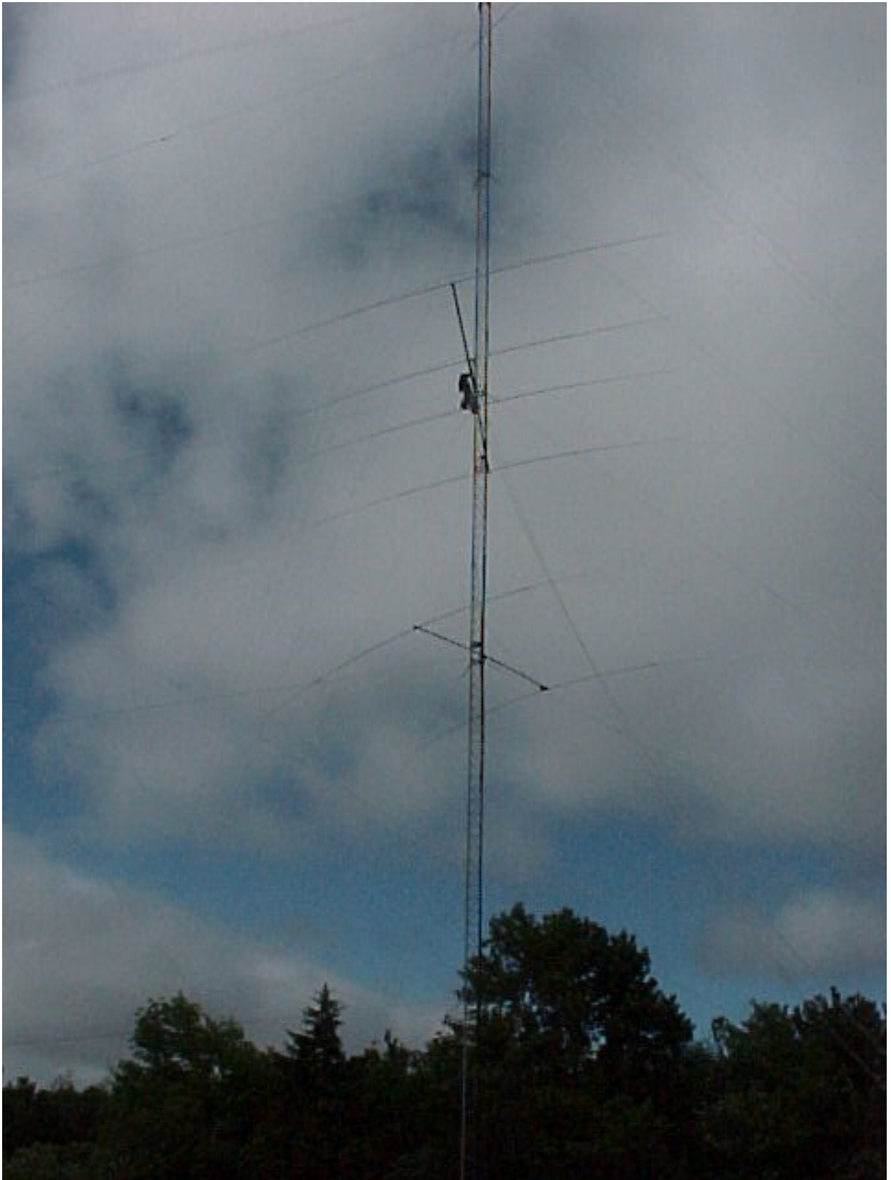
Figure 176 Tip and turn to get past guy wires
