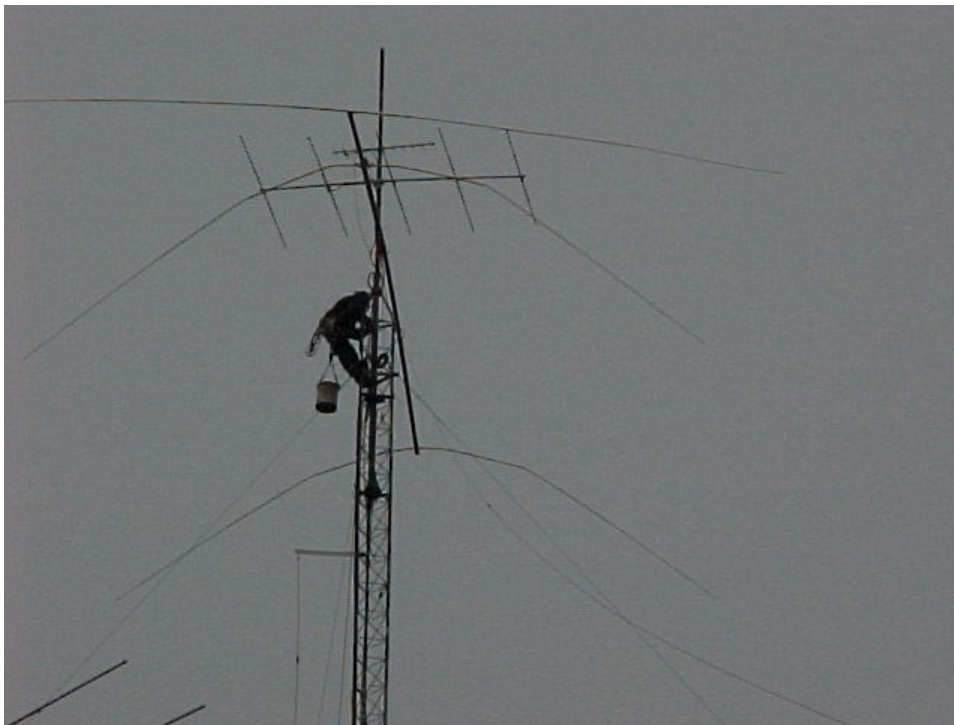
Figure 411 D1 is off and the antenna rotated. D1 is just in the way of tipping and twisting since it is so close to the balance point. So it is taken off first and put back on last.
