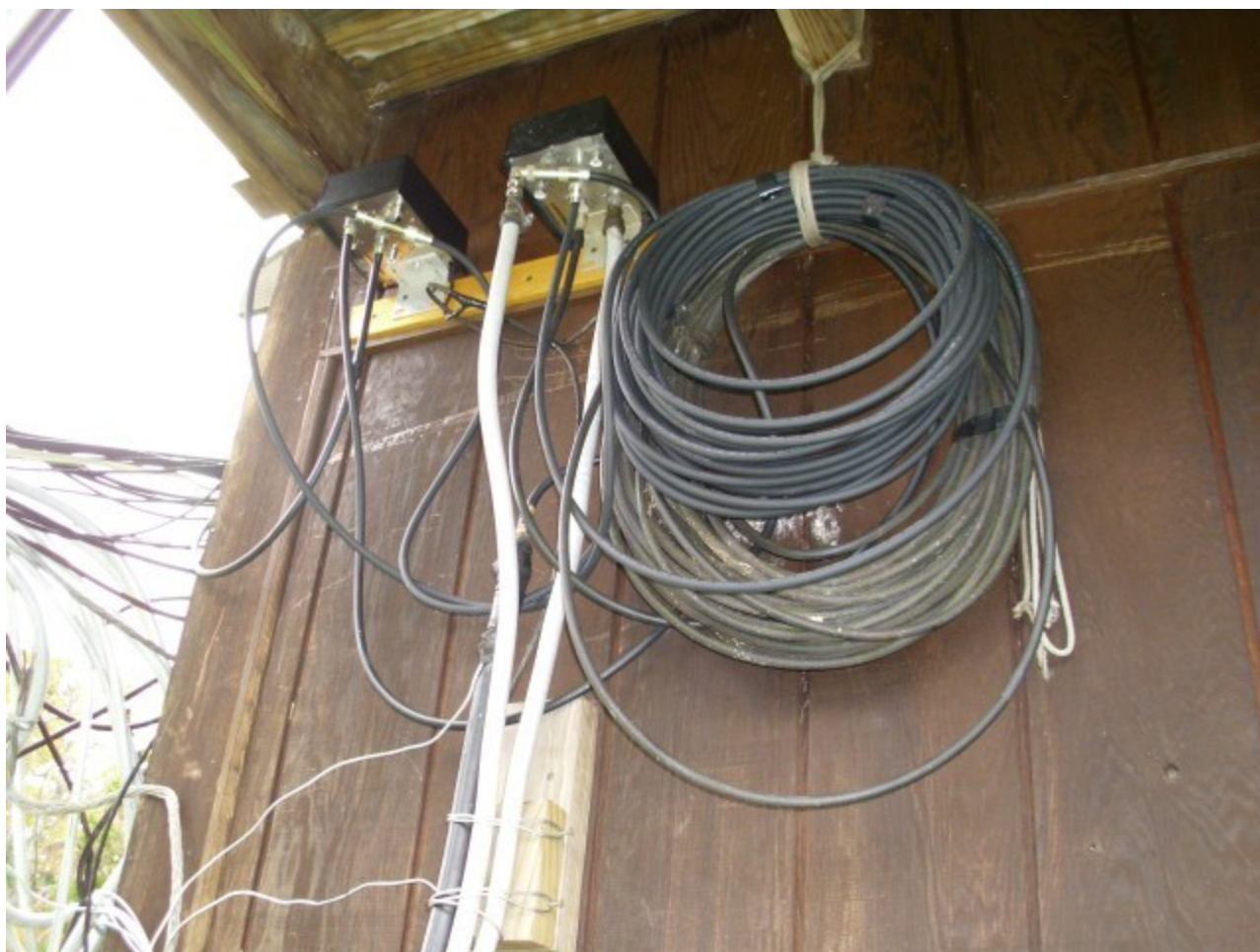
Figure 665 New 160m matching installed
