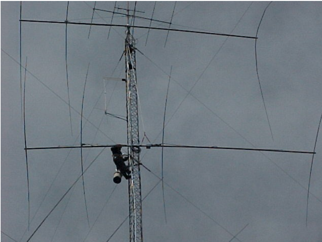
Figure 409 120' 20m4dx just about in place.
