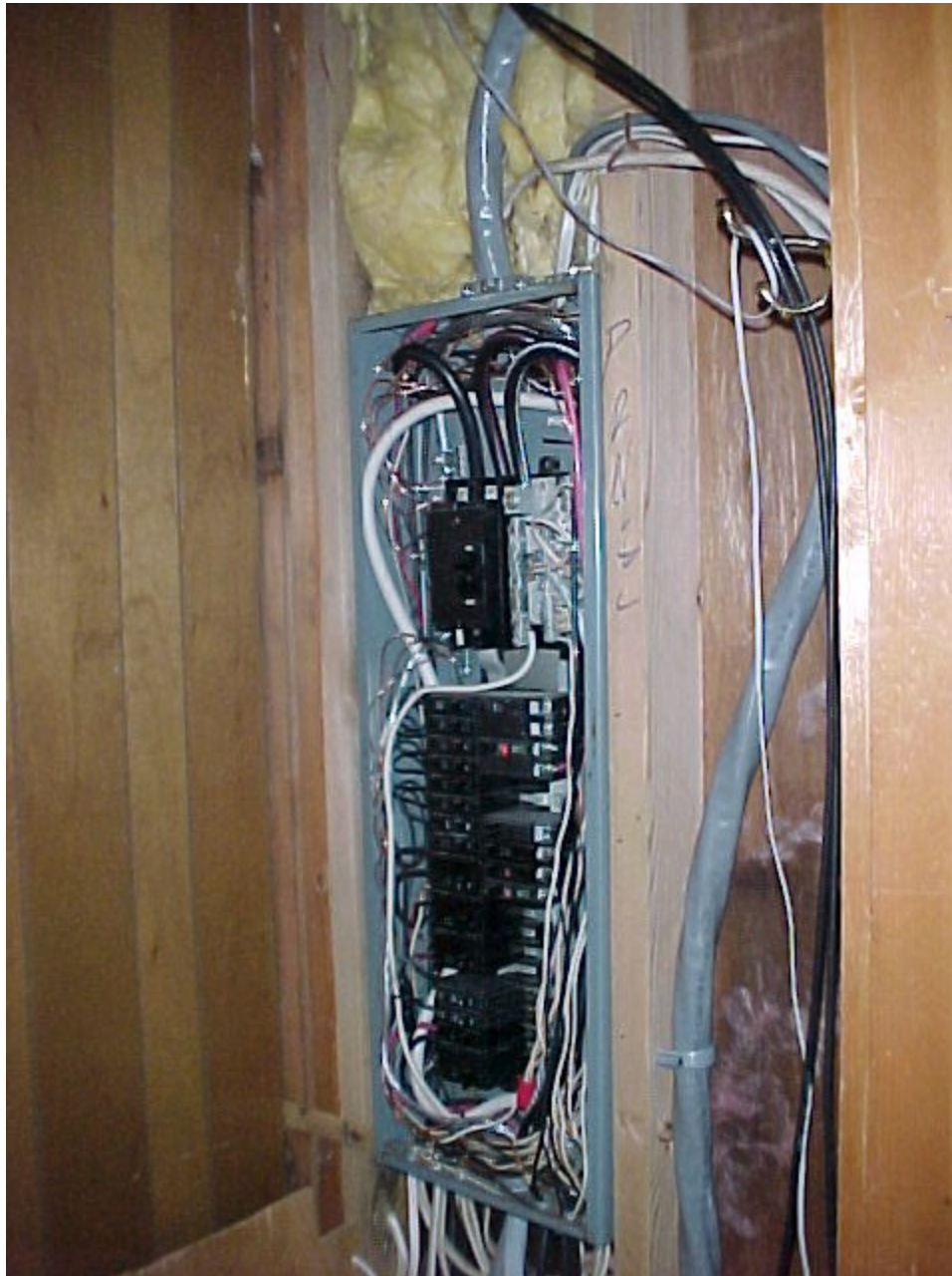
Figure 488 The after view of the main house panel.
