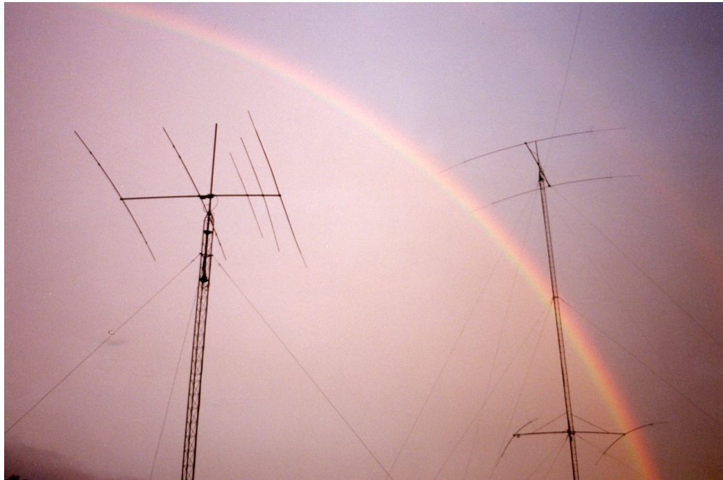
Figure 88 TB5 on temporary tower, 120' 40m tower
