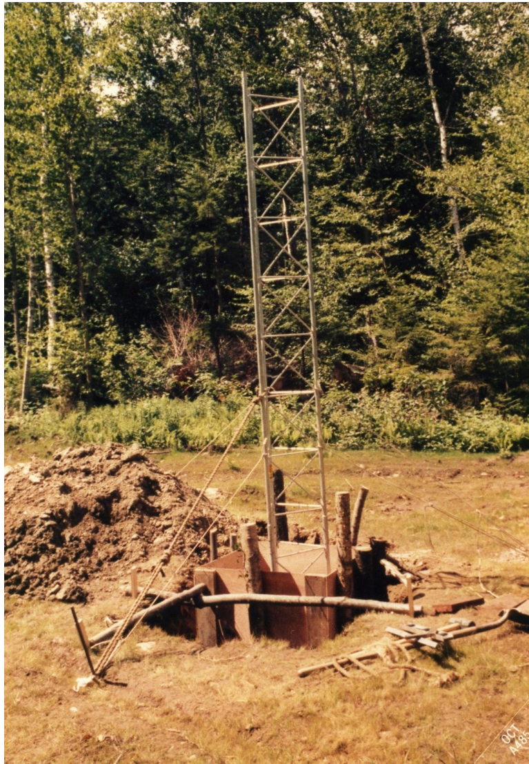
Figure 14 Using one straight section to plumb the base section
