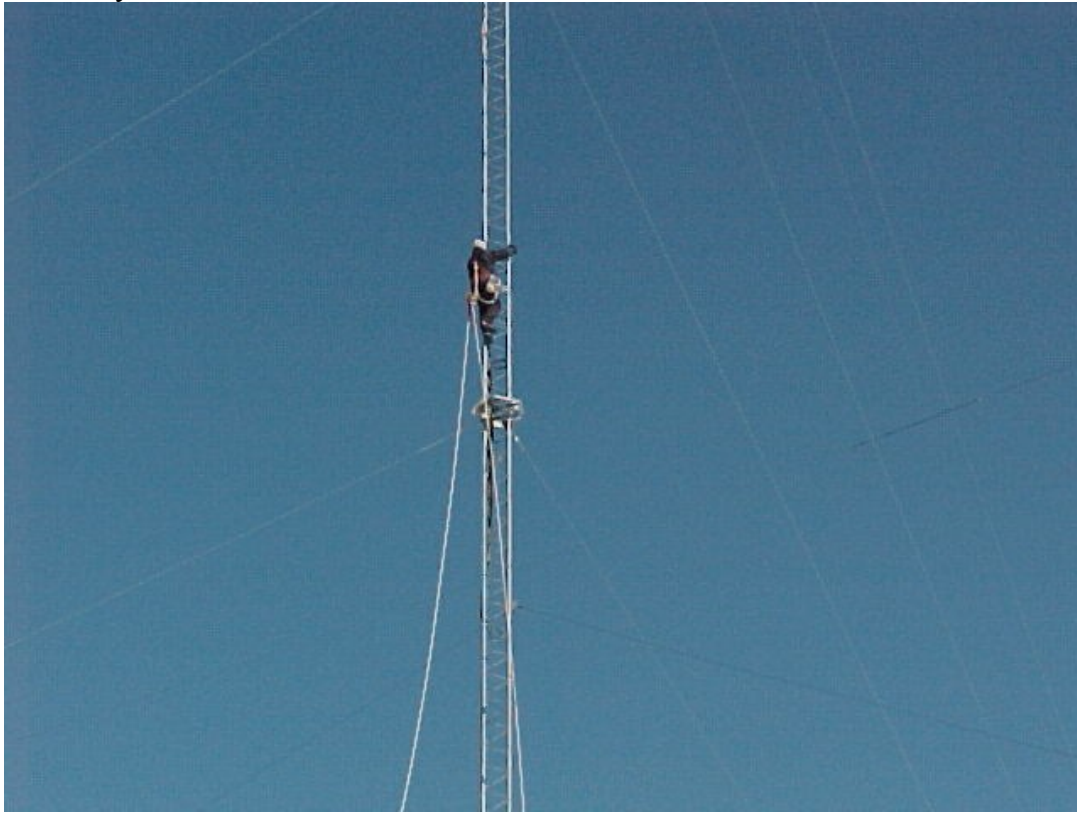
Figure 381 Andrew taking the lifting rope up the tower.
