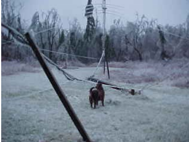
Figure 355 The Beverage post that broke off at ground level
