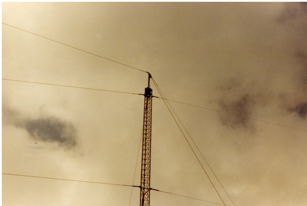
Figure 108 Tram rigged on tower, with back guy in place.
