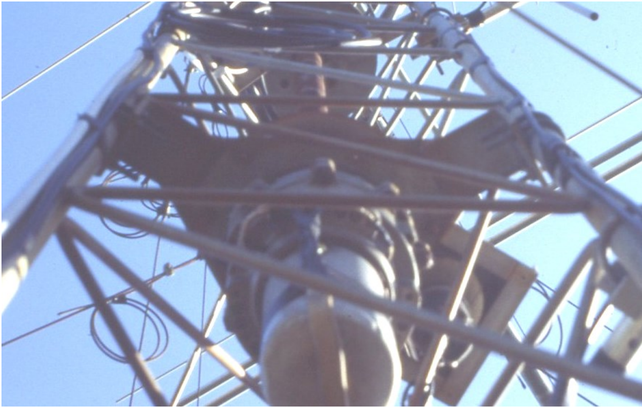
Figure 17 Bottom view of prop pitch rotor with synchro motor on right
