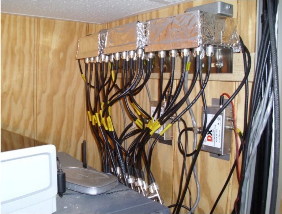
Figure 644 New rx switching installed.
