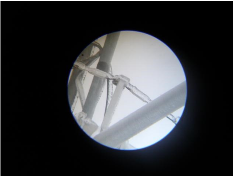
Figure 569 Ice on the 70' 40m4l1dd element truss support.
