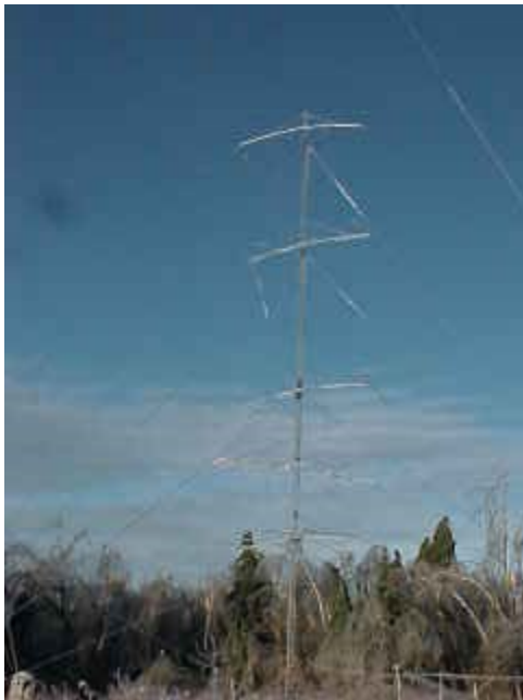
Figure 367 15m tower, a few twisted and broke elements on these.
