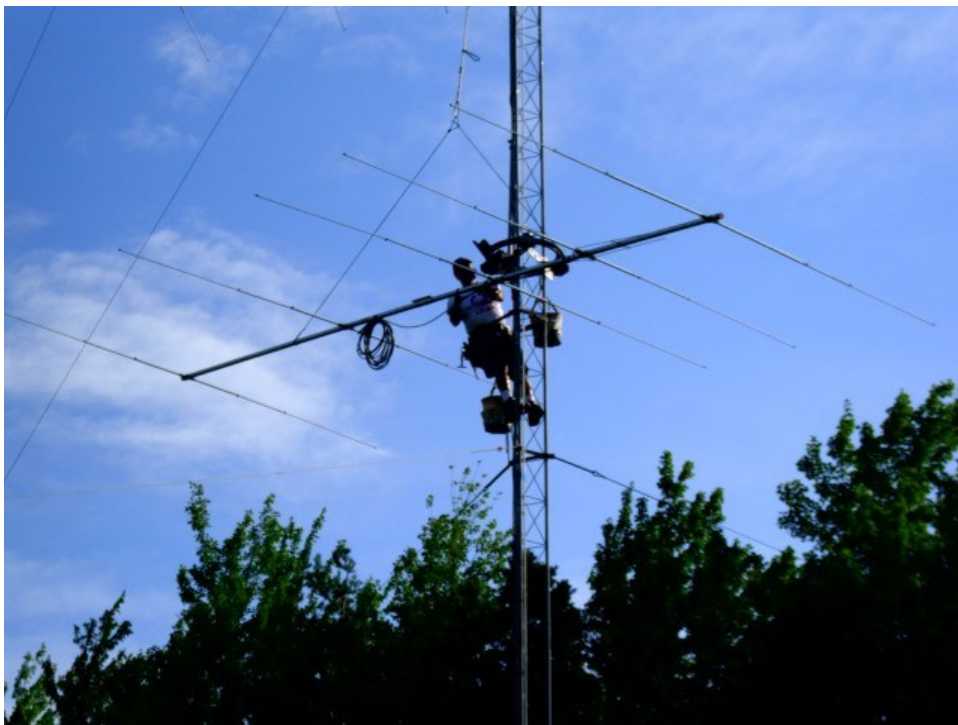
Figure 742 Putting one on ring rotor
