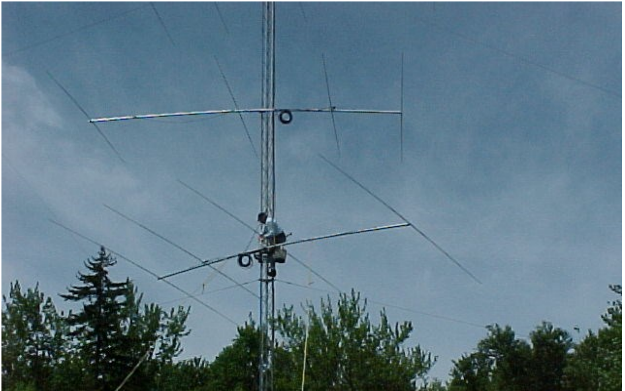
Figure 162 Mounting new 15m in ring rotor.
