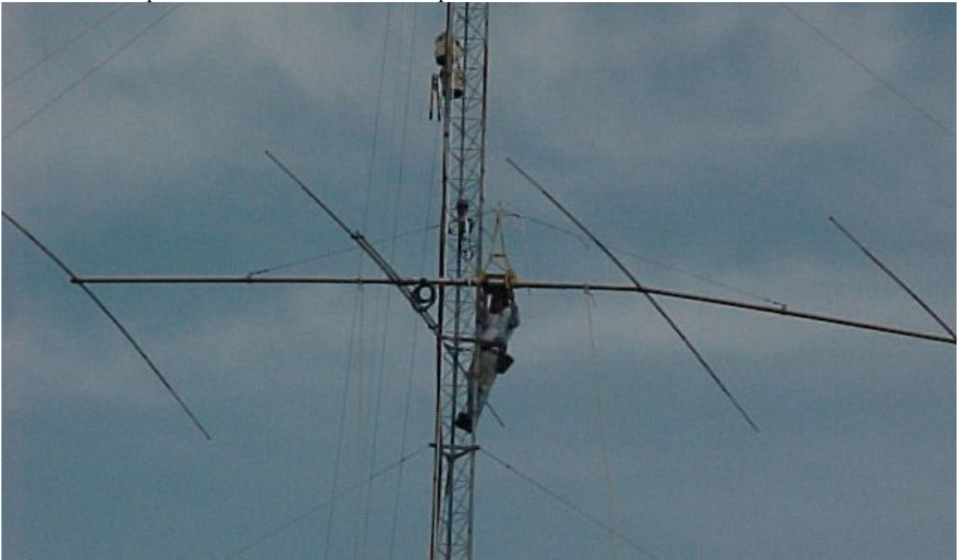
Figure 145 Kinked boom 4 element 20m Telrex rigged to lower.
