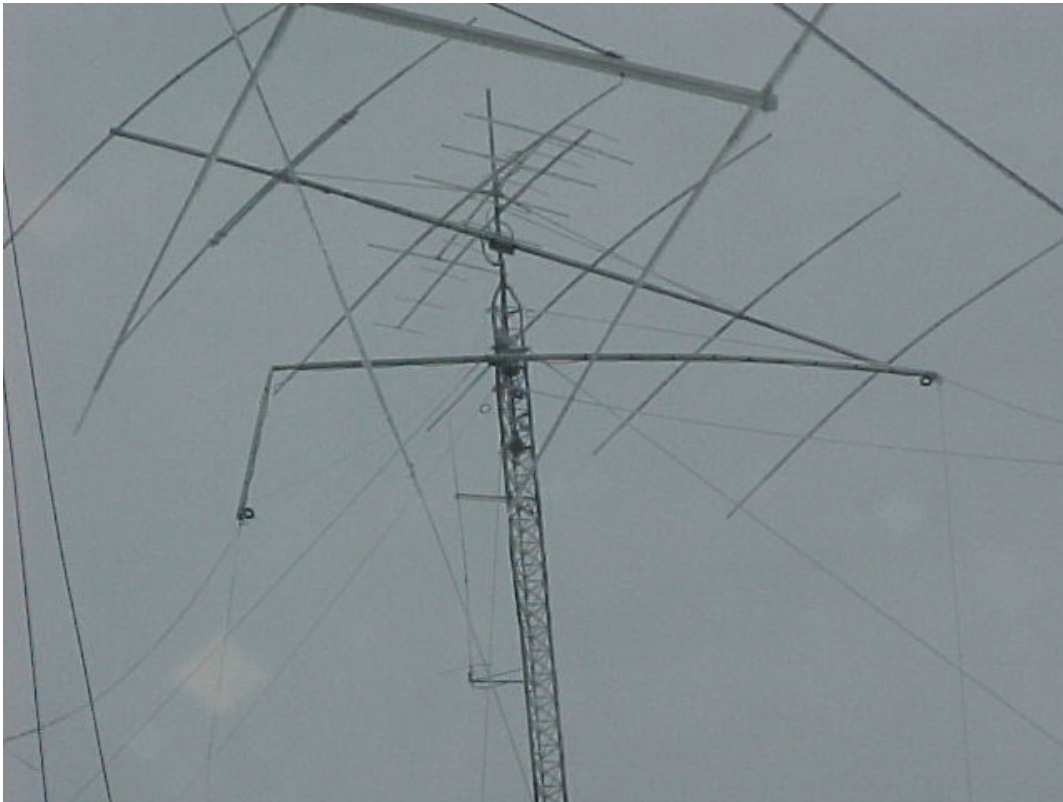
Figure 138 80m beam boom broke.
