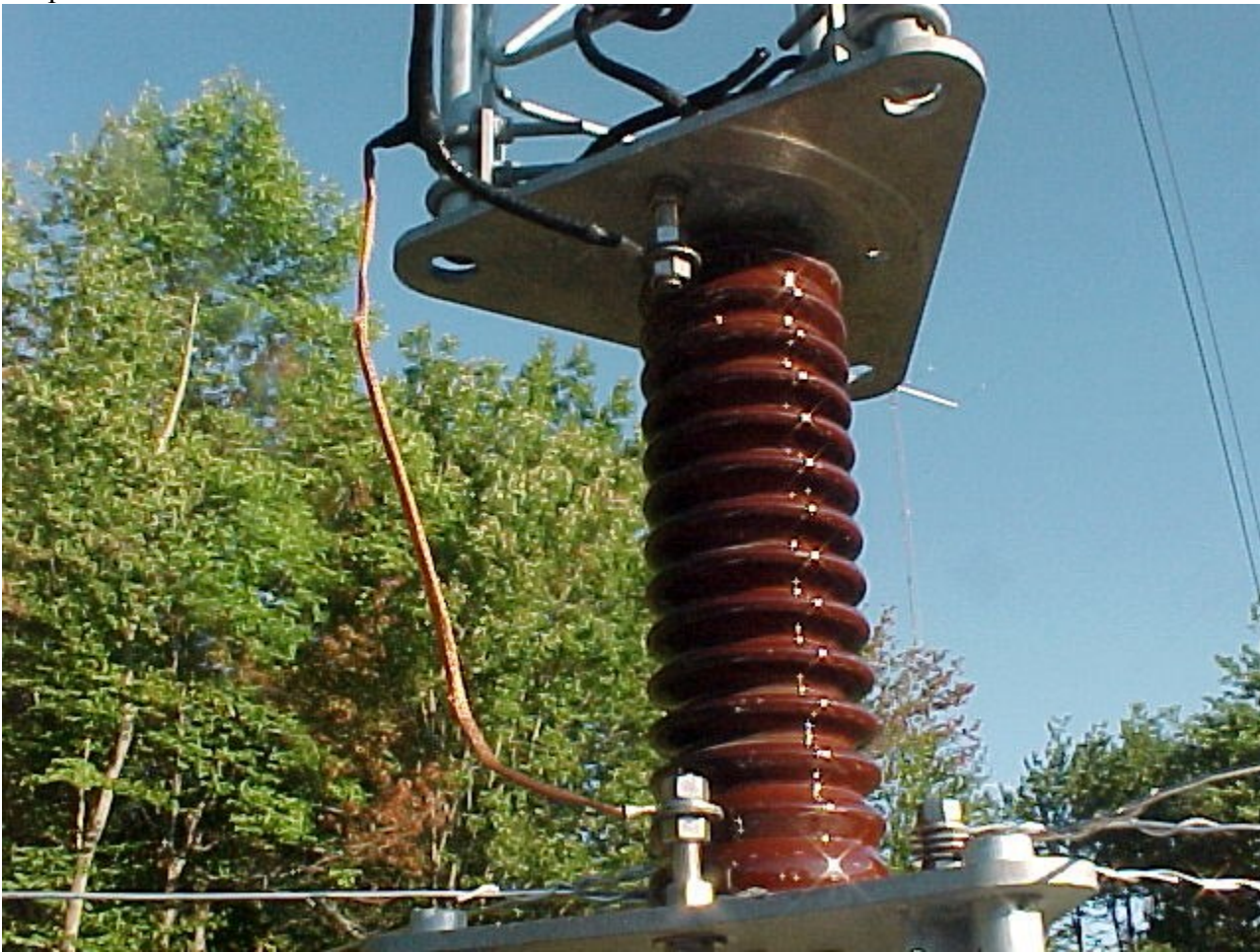
Figure 296 Feed connections.
