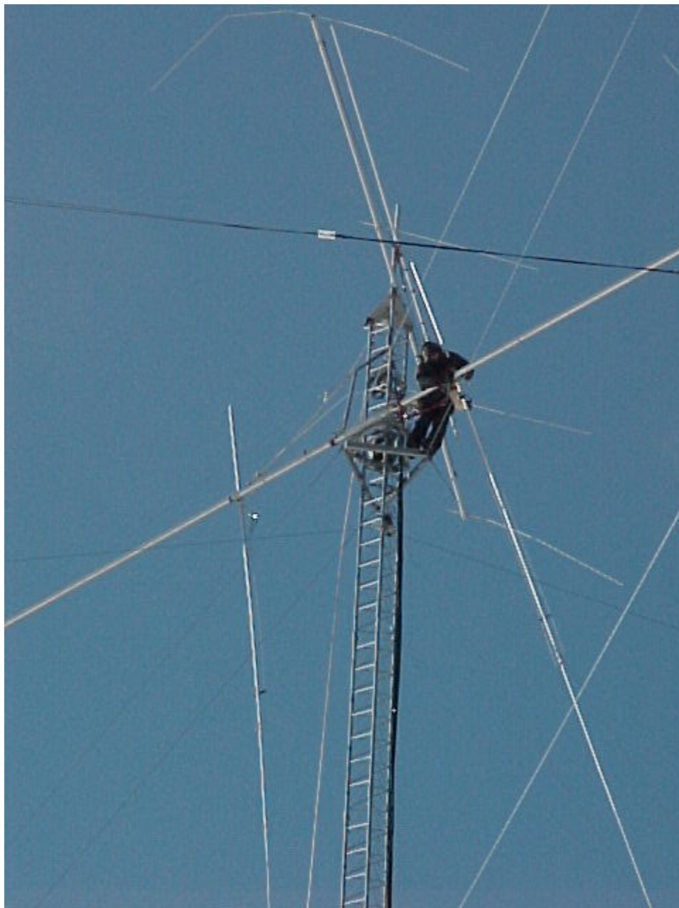
Figure 380 Andrew removing an element on the top 40m.
