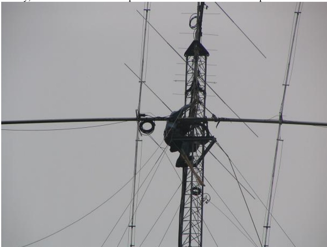
Figure 205 removing temporary rigging.
