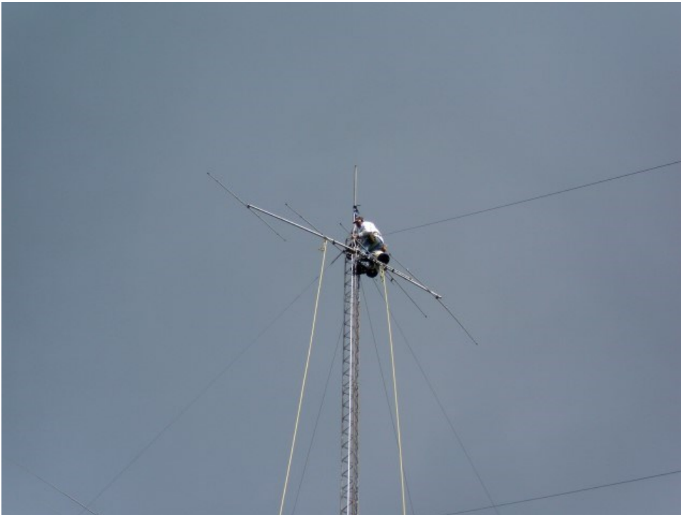
Figure 735 Tilt and Twist to get it under the top guy wire
