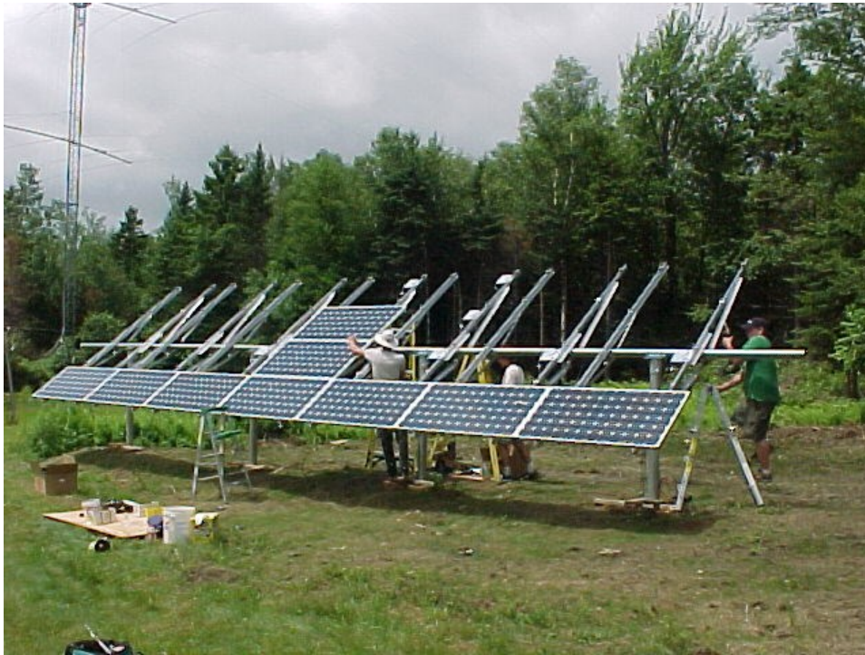
Figure 513 The first panels on the framework.
