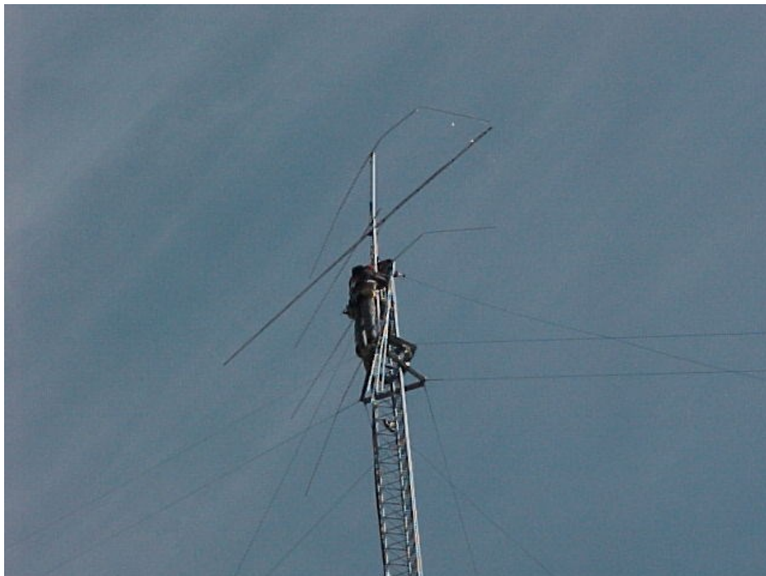
Figure 403 The 10m boom is now vertical and he is replacing elements.
