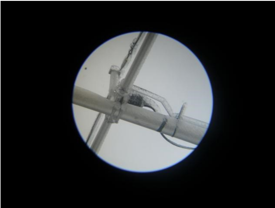
Figure 570 Ice on the 180' 40m4l1dd feedpoint.
