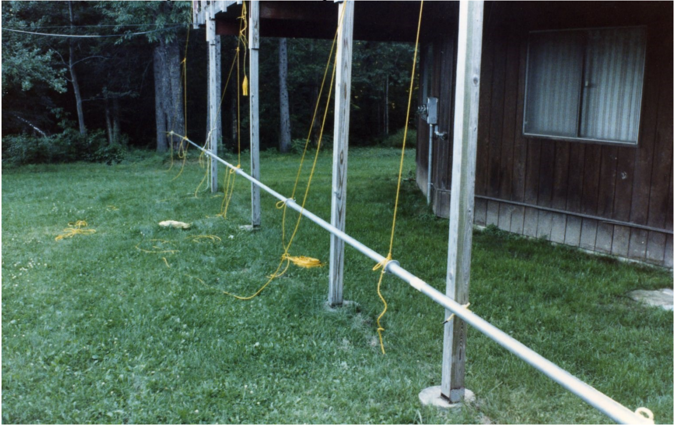
Figure 36 80m vertical of chain link fence top rail
