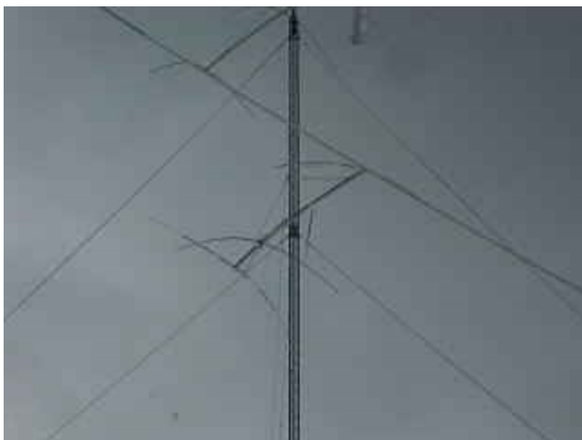
Figure 364 Broke and twisted 15m European antenna at 90'.
