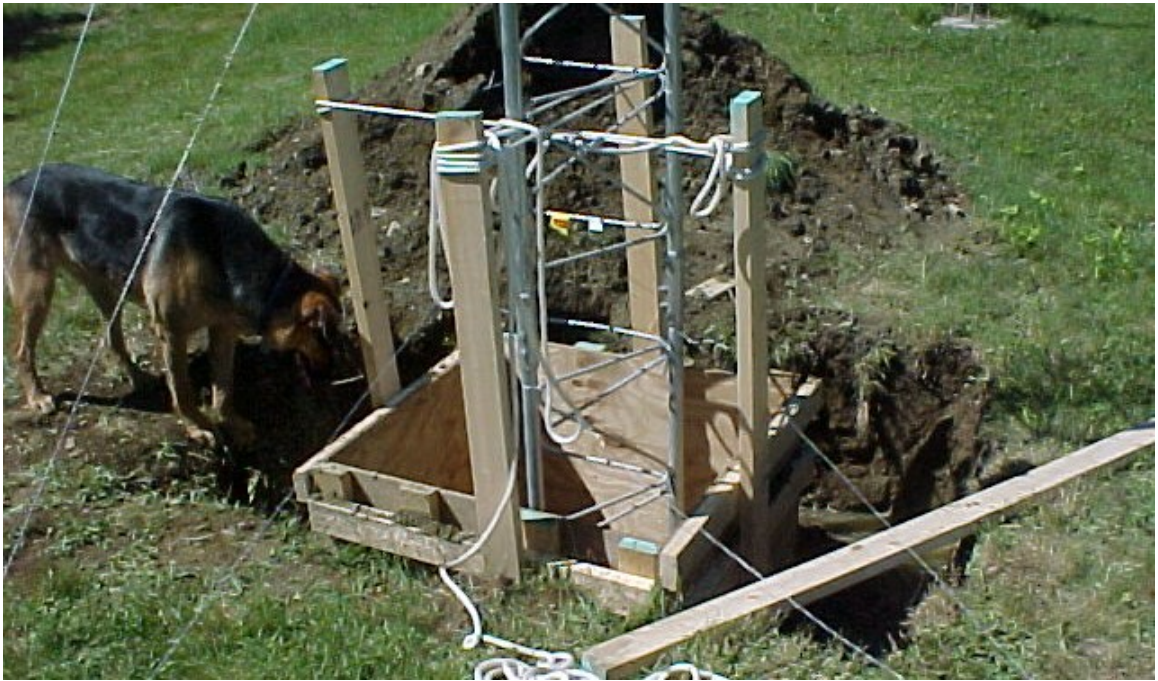
Figure 121 180' base ready for concrete.
