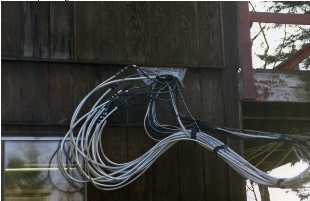
Figure 60 New wall access hole
