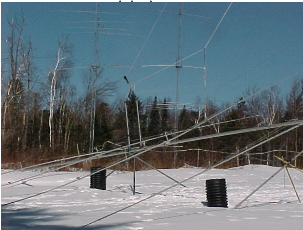
Figure 384 Lift-off, just a bit too much lift on the tipping sling made for a tough start.
