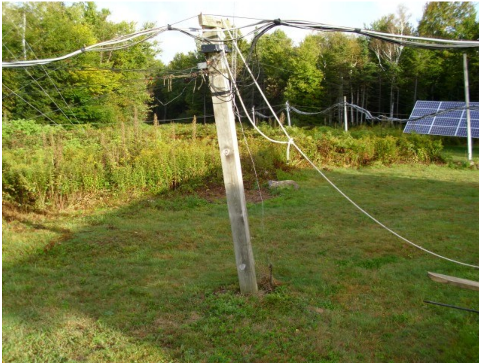
Figure 657 Leaning Beverage pole
