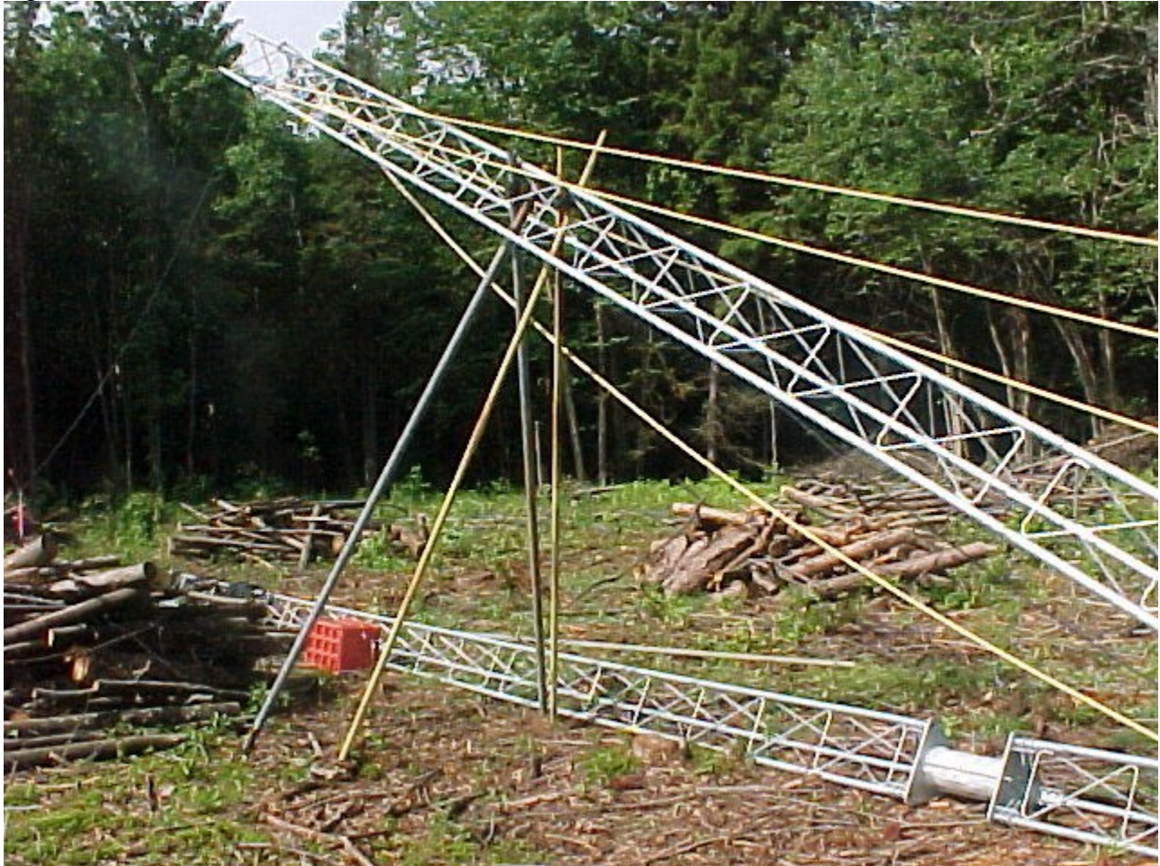
Figure 279 V poles pushing up.
