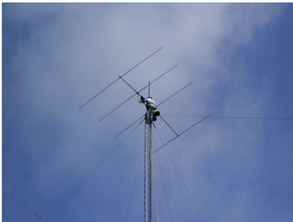
Figure 733 Removing last old Yagi, rigging
