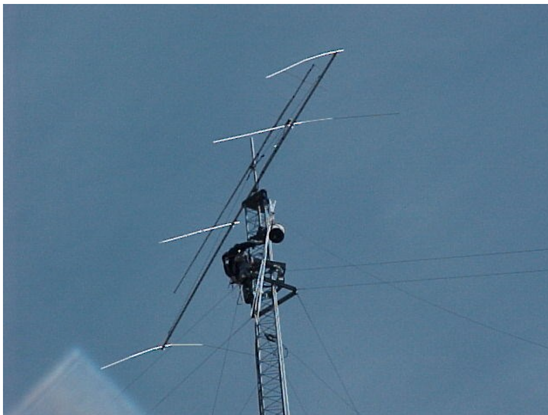
Figure 402 Andrew with new 10m elements getting ready to repair the 180' 10m4dx.
