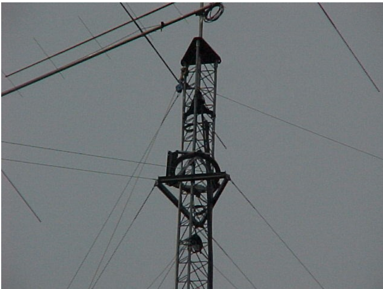
Figure 192 Tram and Rigging in place.
