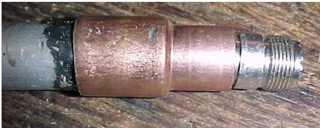
Figure 849 Reducer with barrel connector on CATV hard line
