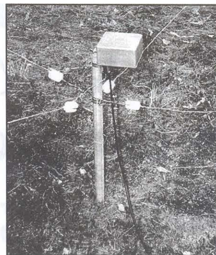
Figure 4—A photo of the central connection point at the base of a two-loop system, as installed at K9AY.
