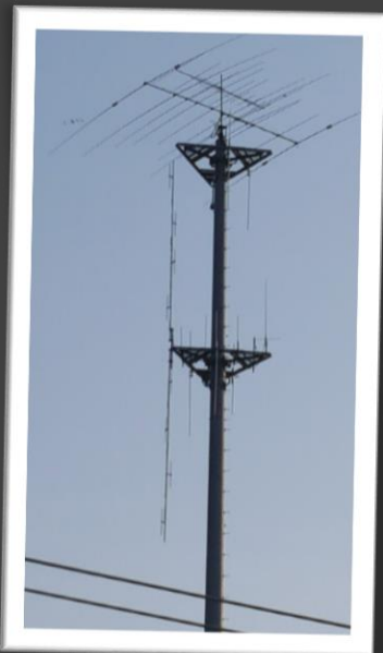
Collins County/Richardson, Texas ESDA Tower with Ham antenna array
