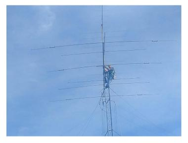
Anyhow, suited up in my shiny new boots and climbing gear and went up and found the driven element U-bolt and saddle had moved somehow and was tilted off level and Steve sent up a small bubble level and I was able to move the driven element back to level and retightened the u-bolt saddle clamp back down snug. Carried my Iphone up there and took some different view photos for Steve to show him what all those birds see when they are gathered on his antenna farm up high.
