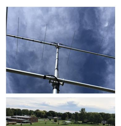
Moved up to the very top of the tower and stood on the thrust bearing flat top plate and moved the 6 meter beam back into alignment with the 2 meter beam and Steve eyeballed the alignment from across the street this time and then tightened the beam clamp bolts back down.
