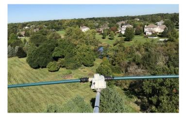
After the ground crew gave the thumbs up on alignment with the SteppIR beam I locked it down in place and Keith and I dressed the coax run coming off the 2 meter beam to the mast pipe and the loop on his other beam.
