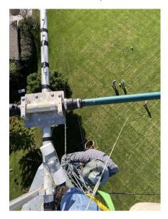
I went up first and got on the very top plate of his 100' tower and belted off around his mast pipe and it was a perfect height for me as I could just look across the top of the mast pipe and it was a piece of cake to mount his beam after he hoisted it up and handed it up to me.
