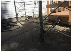
This was a big improvement to my coax runs as they now come off the tower leg and right into a weather head next to the concrete pad and then go underground to another weather head right next to the entrance panel. No more tripping or stepping on coax laying on the ground and now there is just a minimal amount of coax exposed to the critters to chew on and this is coated with a critter repellant that seems to work well.
