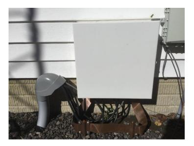
My previous method of getting coax to the radio room was to drill holes large enough to pass the coax and then seal the coax run. So now; the lightning arrestors are not exposed to the weather and much easier to service should something happen. I pulled in extra cords to allow future runs of coax to be added or removed easily when needed.
