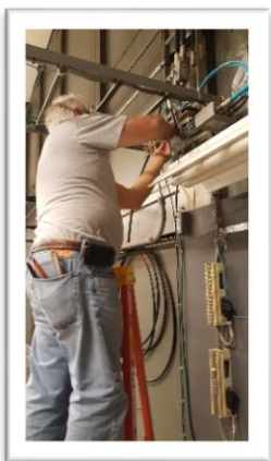
Removing the WX9WX Repeater
