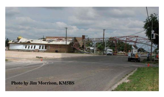
Communication Tower (400 ft.) Down In Seminole, TX Wind Gusts Were Clocked At 98 MPH This Tower Carried The Fire and EMS Antennas Note The Crushed Church
