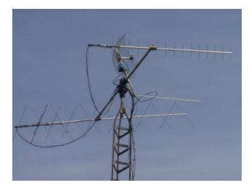
The preliminary equipment for the satellite station consisted of a 16 element cross-polarized beam for 144 Mhz, a 30 element cross-polarized beam for 435 Mhz, a Yaesu azimuth/elevation rotor, and a 2.4 Ghz antenna and 2.4 Ghz downconverter.
