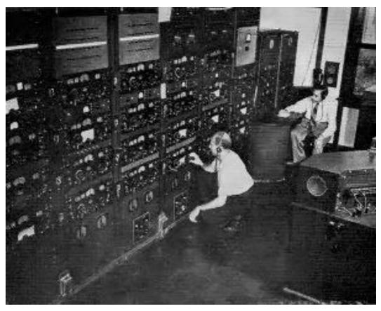
**Figure 126:** A Silver Hill monitoring officer in the foreground adjusts the receiver for a station to be monitored. The officer in the background scans the ether for new stations.
