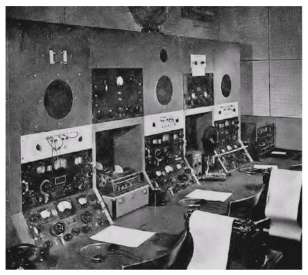
Figure 153: Operating positions in the intercept room at the Allegan, Michigan primary monitoring station circa 1944. Signals were recorded on wax cylinders and paper discs for transcription and analysis.
