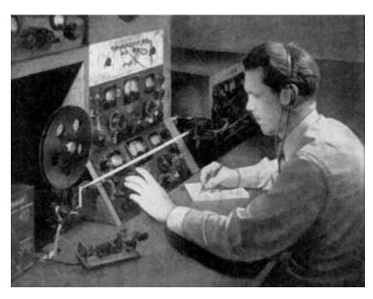
Figure 33: William J. Hoffert (W5HVB) recording high speed code on a Boehme tape machine.
