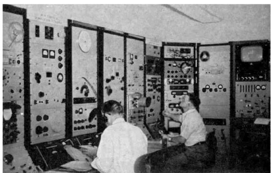
**Figure 179:** Laurel monitoring station interior. Man on left is running a frequency check on an incoming signal. Tape recorders used to record evidence of violations are located in the upper left and right side of the photo. The DF antenna direction indicator is in upper left below the tape recorder. A teletype terminal is located in the lower right.
