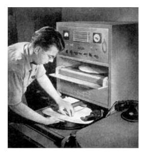
Figure 122: Flexible disk recorders used to record unknown signals for further analysis.
