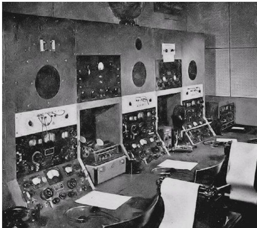
Figure 142: Operating positions in the intercept room at the Allegan, Michigan primary monitoring station circa 1944. Signals were recorded on wax cylinders and paper discs for transcription and analysis.
