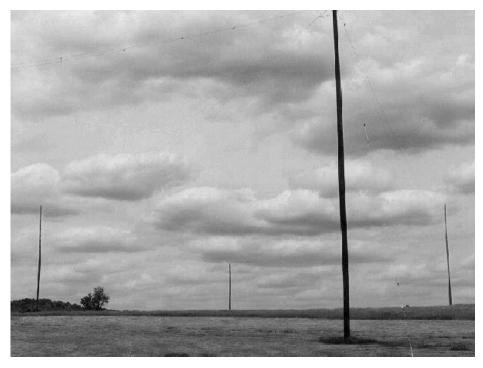
Figure 131: Rhombic antenna installation.
