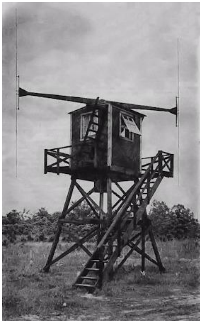
Figure 74: Allegan, Michigan monitoring station Adcock direction finder circa 1944.
