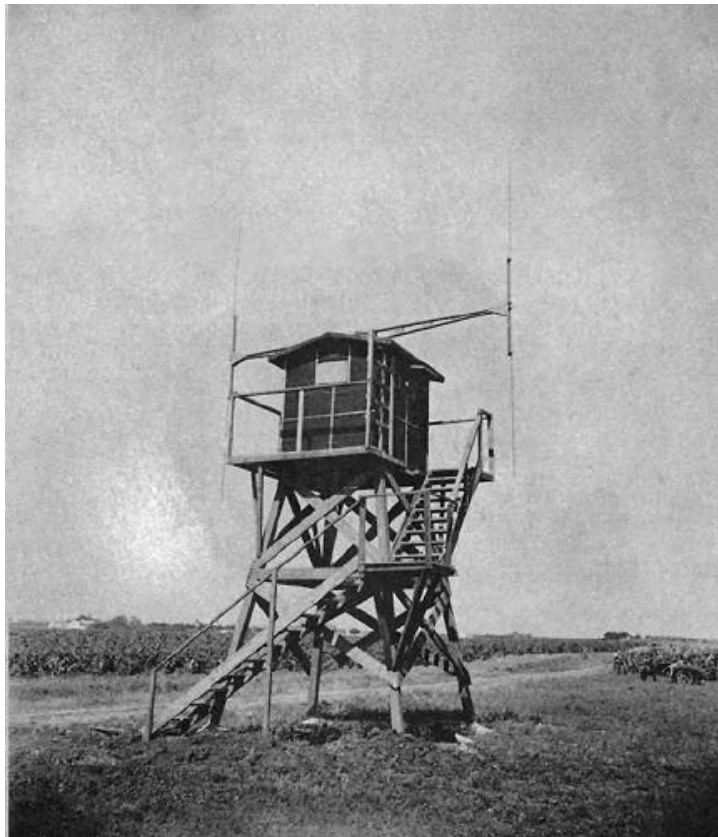
Figure 2: Adcock direction finder at the Scituate, Rhode Island monitoring station.
