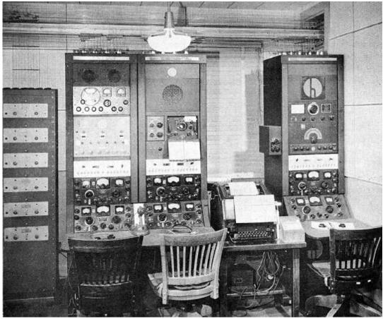
**Figure 83:** Intercept positions at the primary monitoring station in Allegan, Michigan. SX-28s were stacked above another for the convenience of the intercept officer copying both the spy and control station on different frequencies. Transmitters on the left operated on different frequencies to transmit alerts to the secondary monitoring stations and furnish frequencies and calls in FCC cipher code when a case became active.
