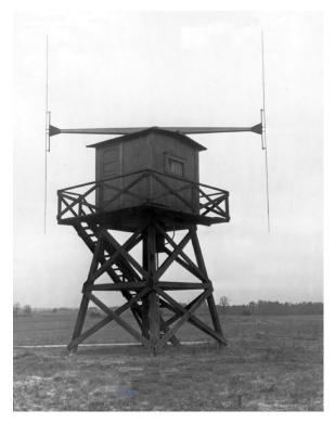
Figure 116: Adcock DF at Scituate, R.I. with improved antenna.
