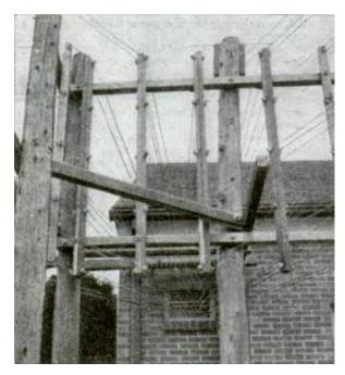
Figure 46: Antenna feed lines entering a monitoring station.
