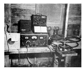
Figure 117: Interior view of Adcock DF shack.
