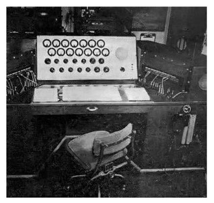
Figure 125: Programs received at Silver Hill were routed through this monitoring console.
