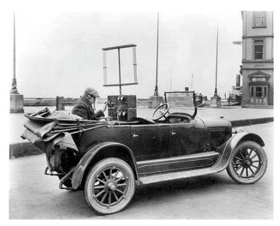
Figure 1: Experimental DF Mobile Unit.
