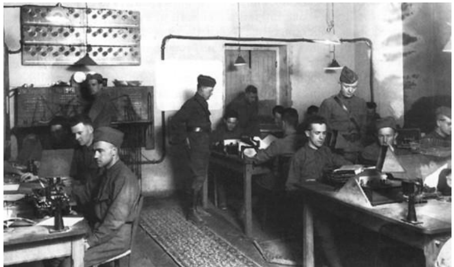
Figure 17: The radio room at Chaumont
