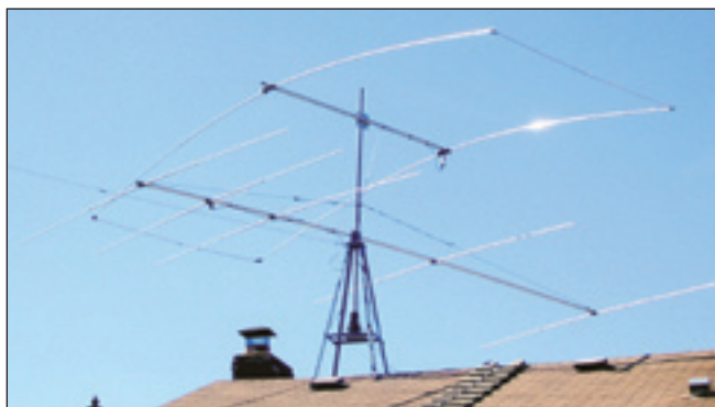
Figure 10 — Moxon mounted on the HF roof tower above the five element 10 meter beam. The roof ladder shown helps save the shingles and enhances safety.
