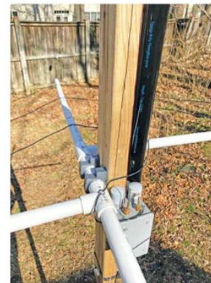
Figure 3 — The spiral wire was secured with cable ties at each corner, and the inside end was connected to the balun. The vertical wire connects to the other output terminal of the balun.
