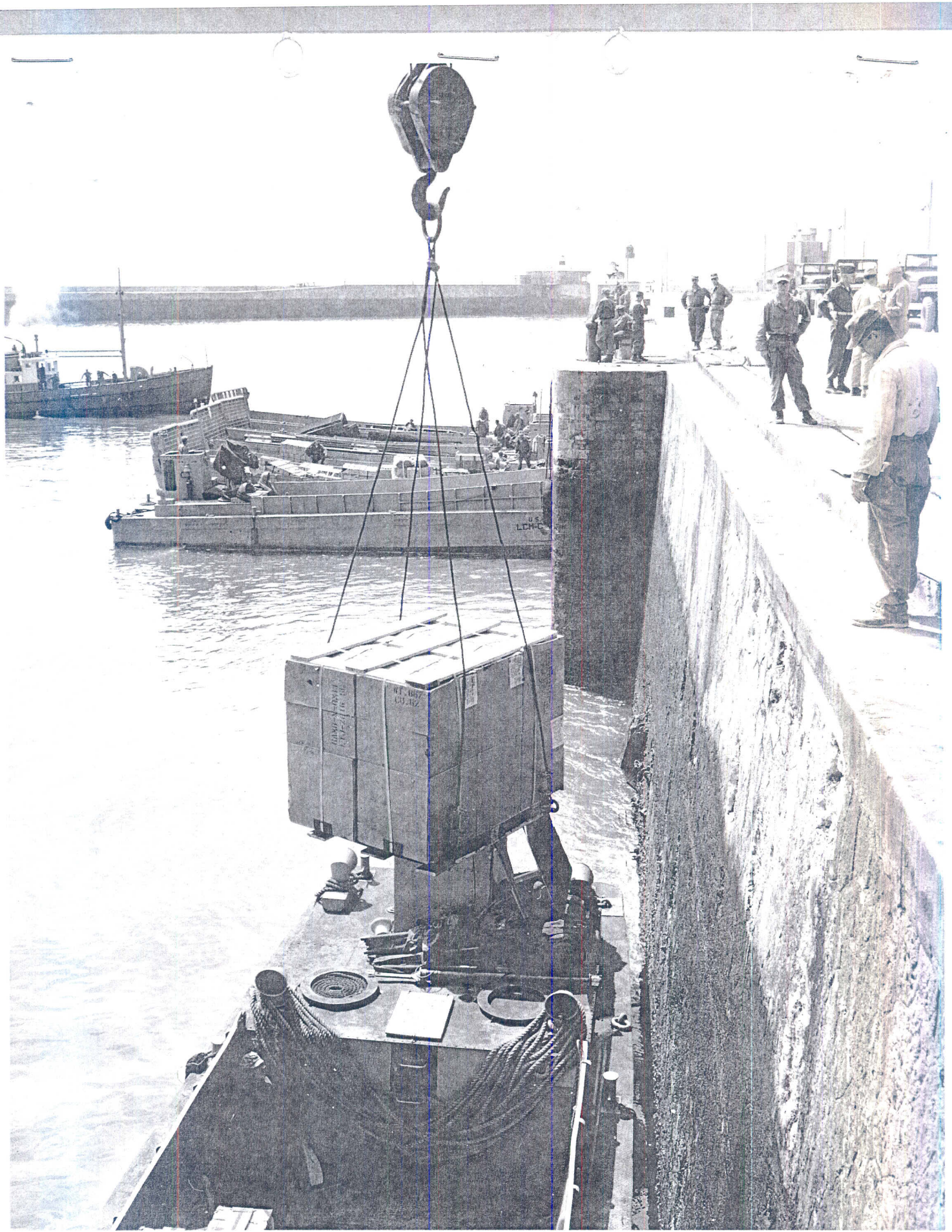
Discharging light OM pallet from LCM at Quei de Maree. LCM's waiting to be discharged were moored where shown and were brought to the discharge points as soon as an empty LCM pulled away.
