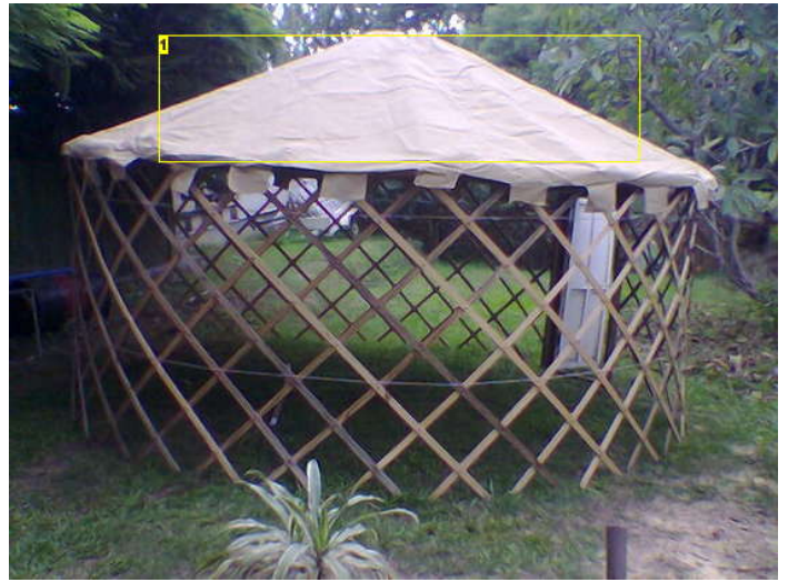
Image Notes 1. loosely fitted roof canvas. (outside view). still a bit crumpled, but this comes out quickly.
