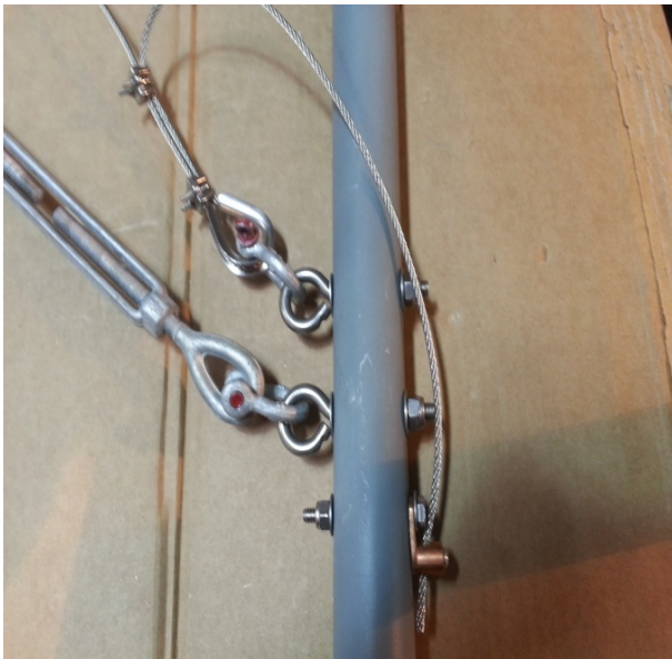
Figure 4-1 879998 Antenna Element with Termination Load
