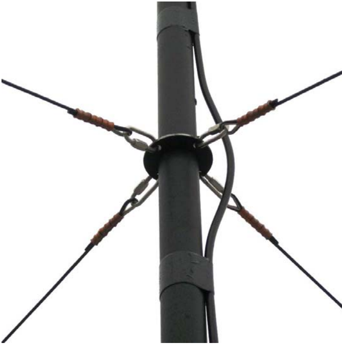
Figure 1-6 Guy Ring Installation
