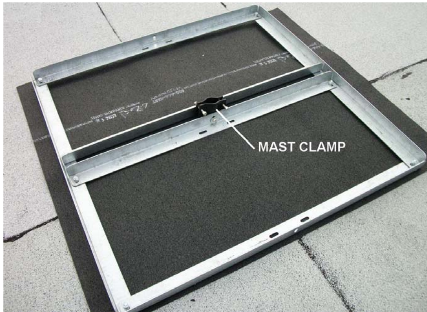
Figure 1-2 Mast Sled Installation
