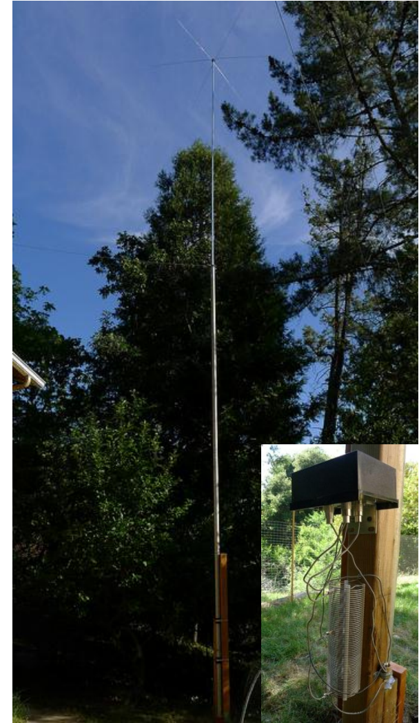
Increased 33' vertical to 45' w/six 5' top hats, added Switchable Base LC's 30
