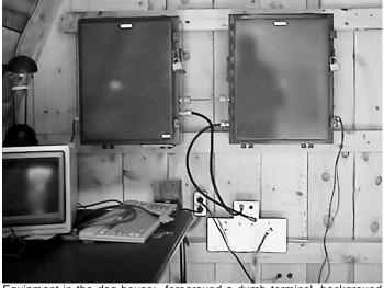
Equipment in the dog house: foreground a dumb terminal, background (left) Corry node equipment cabinet and (right) Corry2 equipment cabinet. Below cabinets is a grounding plate and lightening arrestor.
