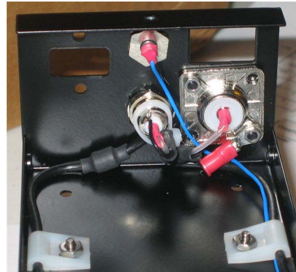
RF IN RF OUT and PTT Wires
