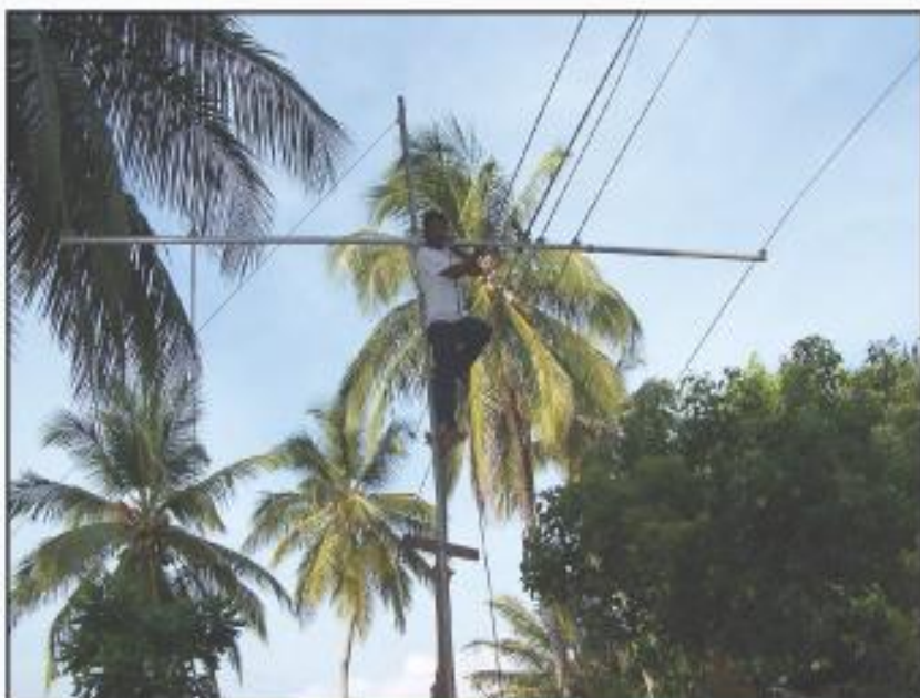
Mr. Madhu, VU2UWZ installing 7 Element Yagi Antenna
