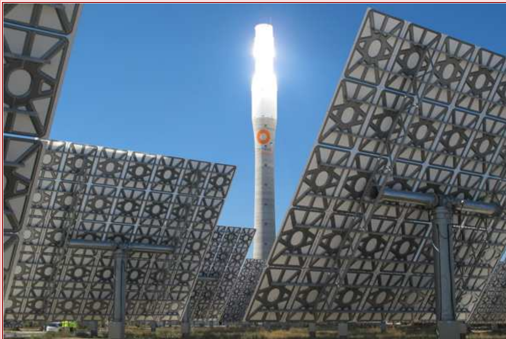
Heliostats & Tower, Torresol Energy, Spain
