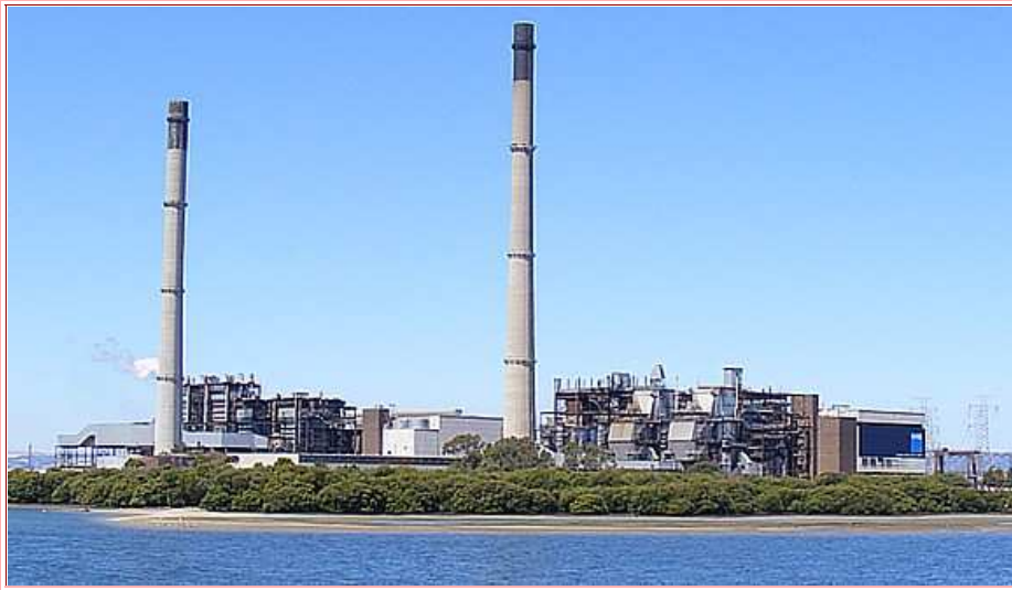
Photo 1 Torrens Island Natural Gas/Fuel Oil Steam Power Station
