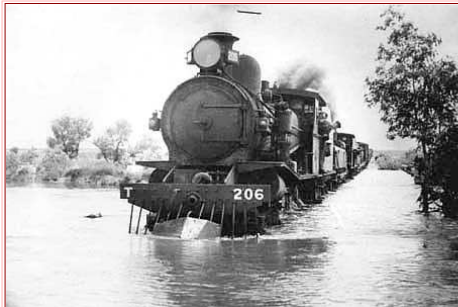
Early Ghan Steam Train moving through flooded rail track
