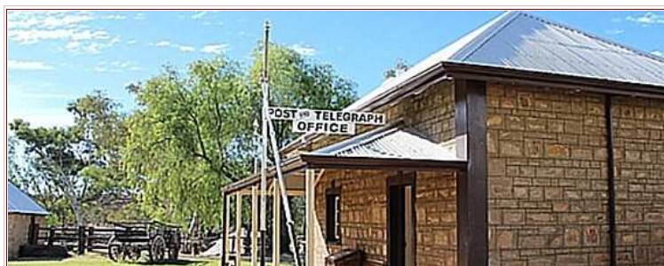
The early Alice Springs Post & Telegraph Office, rejuvenated to restore its original appearance
