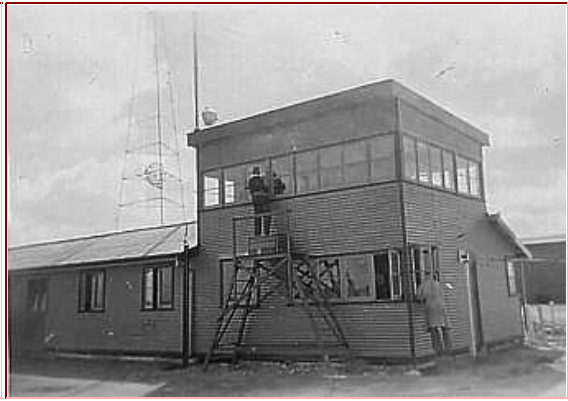
Mt Gambier Aeradio Building
