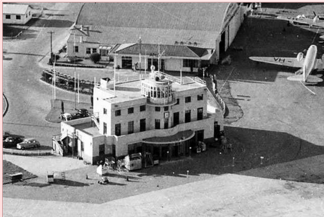
Parafield Control Tower
