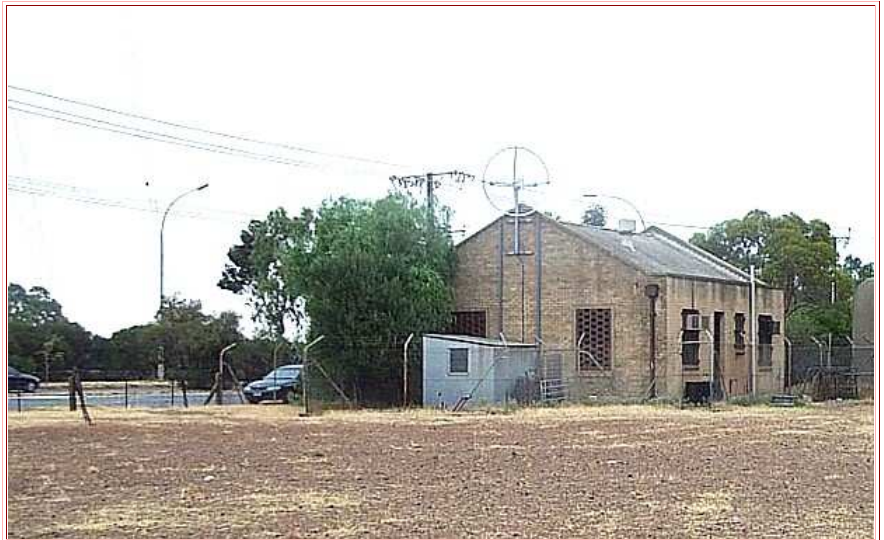
Transmitter Building 5AD & 5KA at the Cavan Photo courtesy of Craig Marich - Chief Engineer
