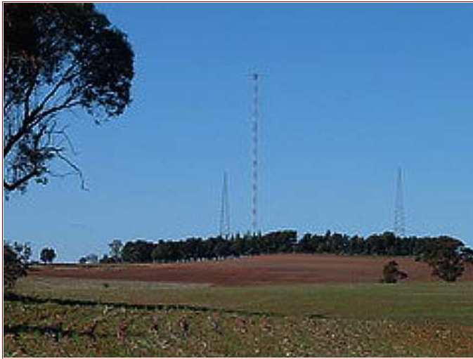
Aerial Towers at SCK including 190 metre tower added
