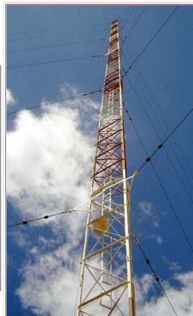
86 Metre Mast used by 5AD and 5KA Cavan Road, Gepps Cross
