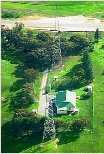
Station SCK at Crystal Brook with original towers
