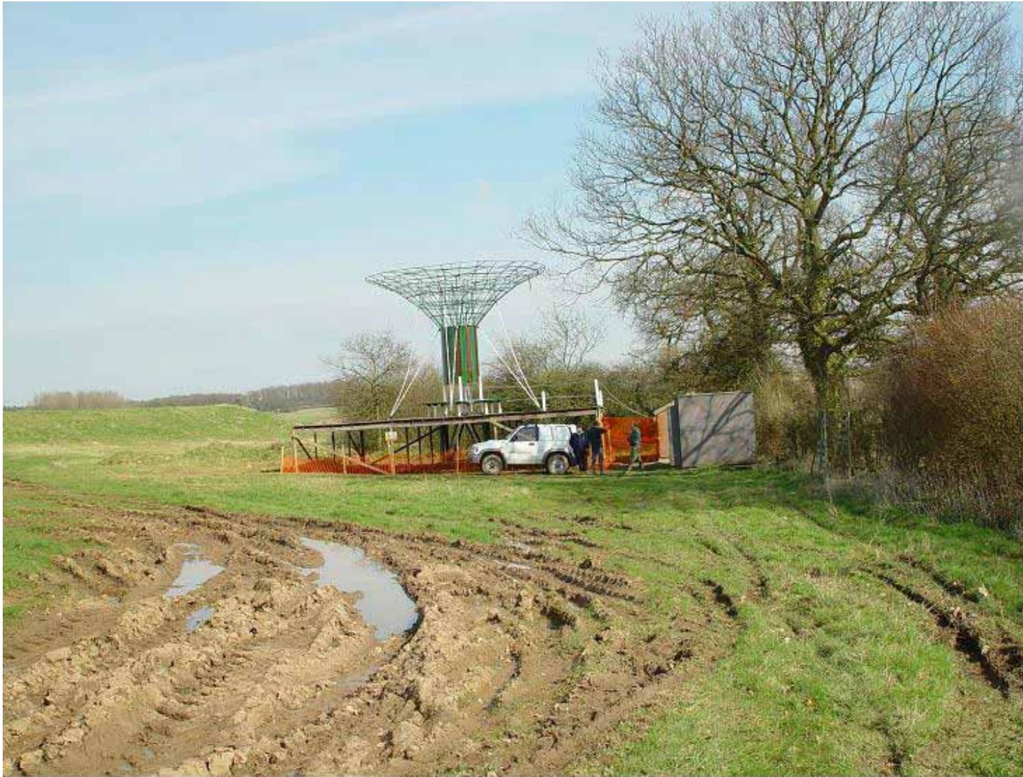
Note: reservoir at left possibly leaking to give wet ground at front: oak tree on right higher than top of CFA; and raised ground-plane immediately under the ‘D-plate’ disc.
