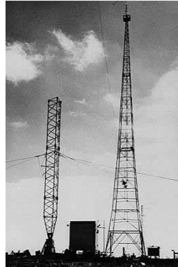
*KNBC (KPO)'s present 550 ft. tower was completed in 1949. This type of antenna is called a Franklin antenna, a design used by only a few AM stations in the U.S. The antenna is easily recognized by the porcelain insulator in the middle of the structure.*
