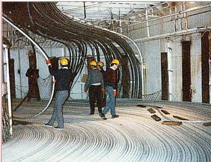
Loading Cable on board CS Cable Venture for ANZCAN project
