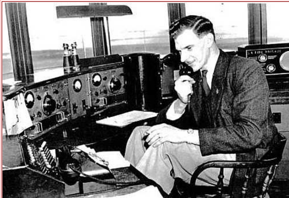
Photo 11 - Parafield Control Tower in Operation 1941 Note the Kingsley AR7 MF/HF receivers. VHF was not installed at Parafield until 1949 (Photo - Air Traffic Control site, ref. 17)
