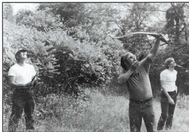
Figure 8.48 — There are many ways to get an antenna support rope into a tree. These hams use a bow and arrow to shoot a lightweight fishing line over the desired branch. Then they attach the support rope to the fishing line and pull it up into the tree.
