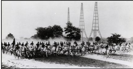
1912: US Navy built "Three Sisters" radio towers. Shown behind US Army cavalry drill at Fort Myer, VA.
