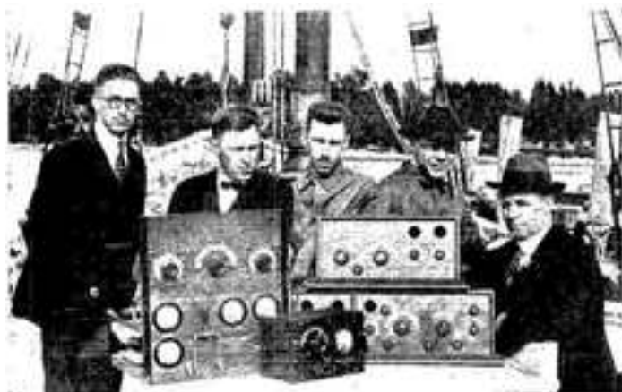
ON BOARD THE "BOWDOIN," AFTER UNPACKING THE EQUIPMENT from a mountainous pile of packing cases. Left to right, F. H. Schnell, ARRL Traffic Manager; D. H. Mix, WNP's operator; K. B. Warner, Editor of "QST"; M. B. West, Goetz engineer who designed the installation; and Dr. MacMillan, the "Bowdoin's" skipper.
