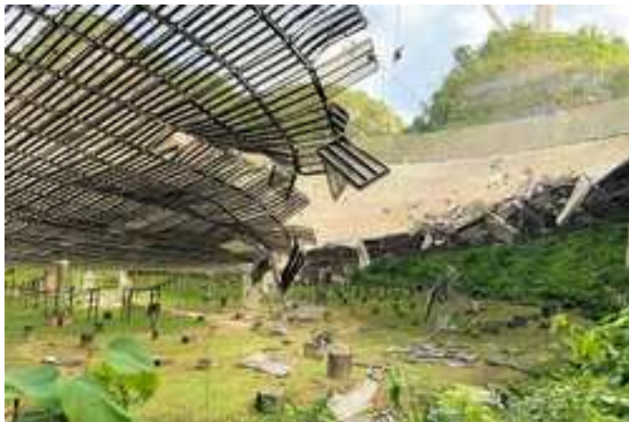
The main collecting dish at Arecibo is among the world's largest single-dish radio telescopes. The reflective dish is 1,000 feet in diameter, 167 feet deep, and covers an area of about 20 acres.
