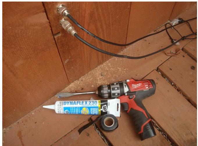
For now a 2m/440 antenna was attached to one connector and a G5RV jr (40m-6m) to the other. Silicon tape was used to seal the connectors because it is easy to remove for future antenna projects.
