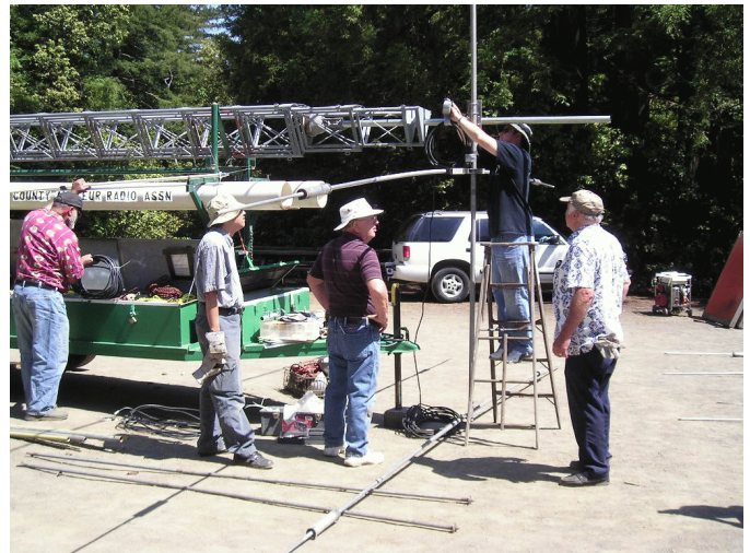
Preparing to install the beam antenna on the trailer-mounted mast.
