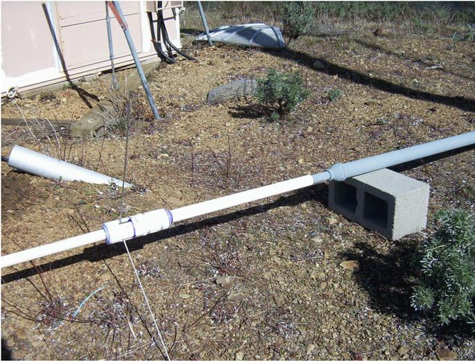
**There's the final assembly—the 1" base mount pipe threaded into an adapter to the 2" pipe mast. The PVC armor now extends down nearly three feet over the pipe—this should provide enough leverage so it won't need to be guyed farther up.**
