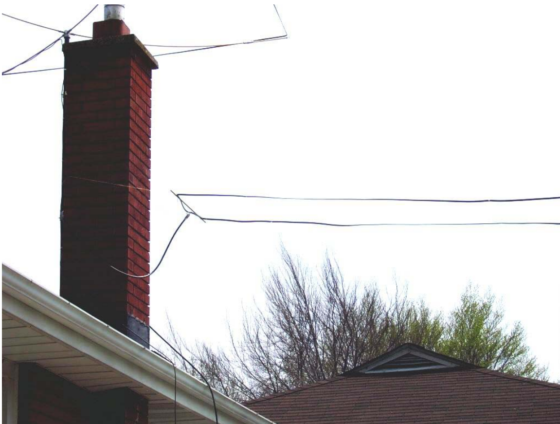
Figure 8e – Feed end of array with coax going directly to the operating room. Above the chimney is a 21 MHz uniform current loop also described in this article.
